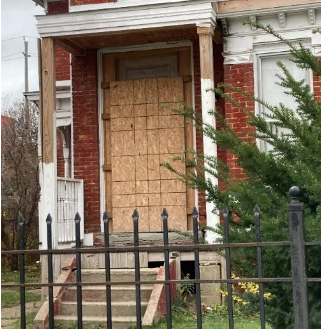
Front porch, current conditions. Photo by staff, 11/25/2024
