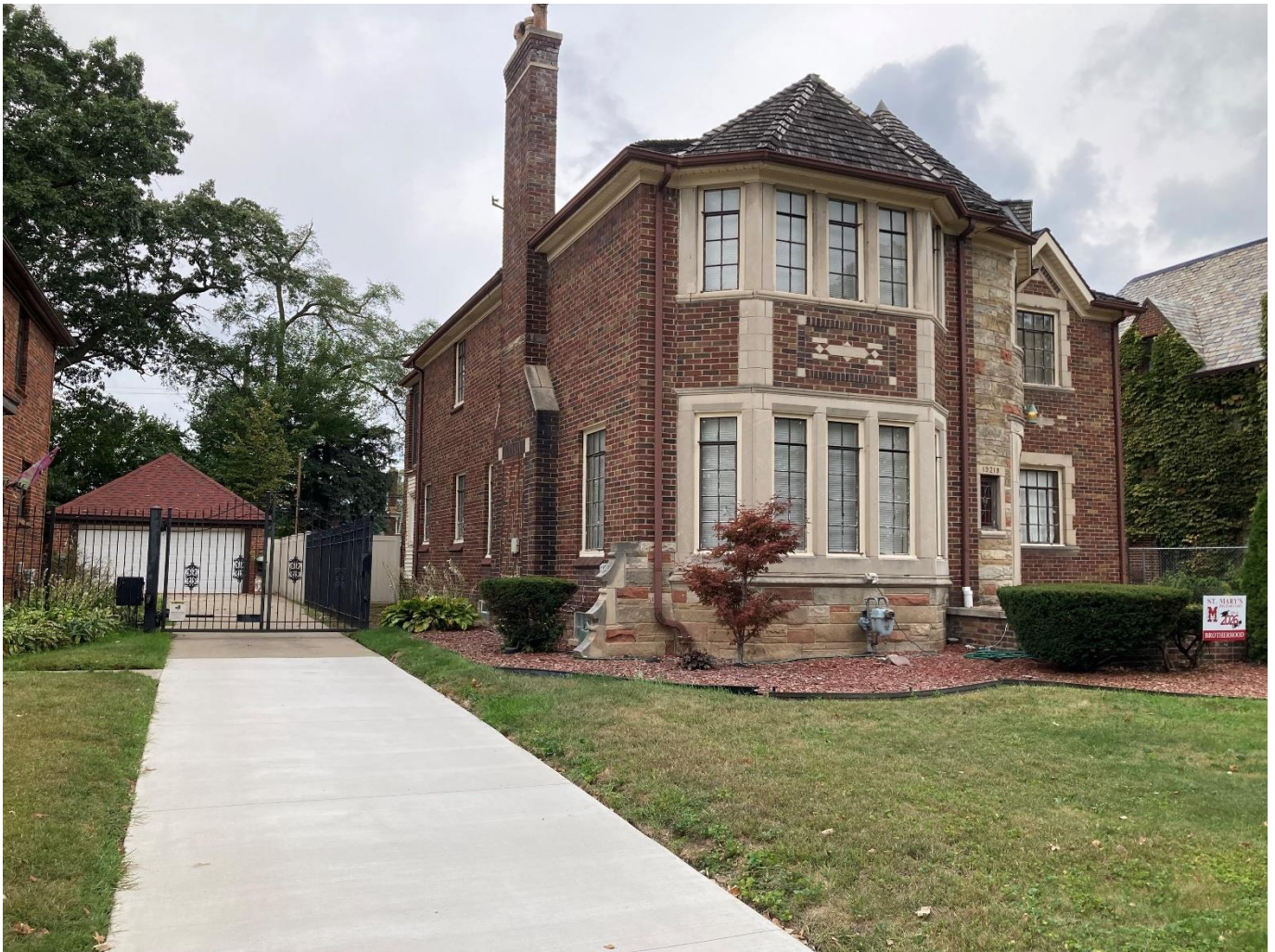
19219 Warrington Drive, south side, along with some of the house's east façade as well. September 2025, staff photo.
