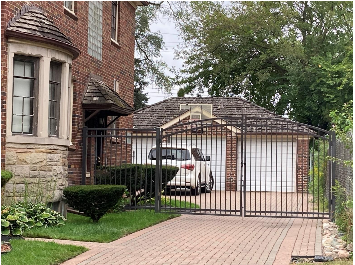
19219 Warrington Drive, north side bay window and side door elements and garage's east side, September 2025, staff photo. Wood shingle roof evident.
