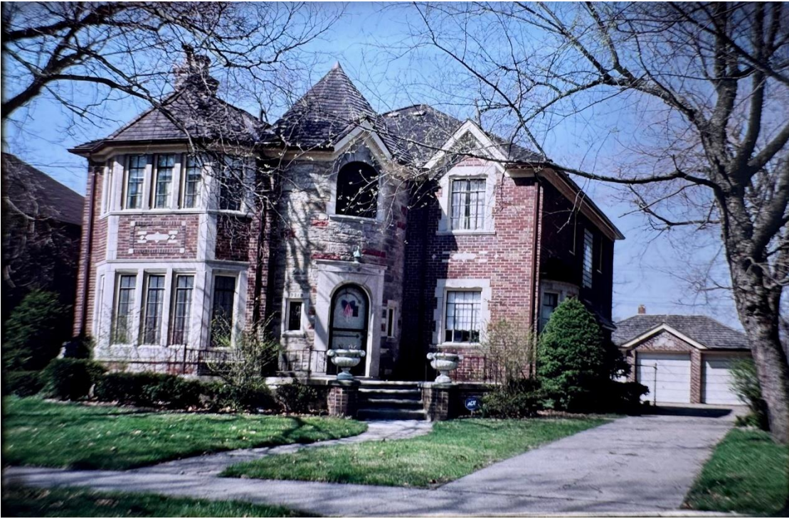
19219 Warrington Drive, Sherwood Forest, Designation Photo, 2002. Wood shingles were on the house and garage at the time of designation.
