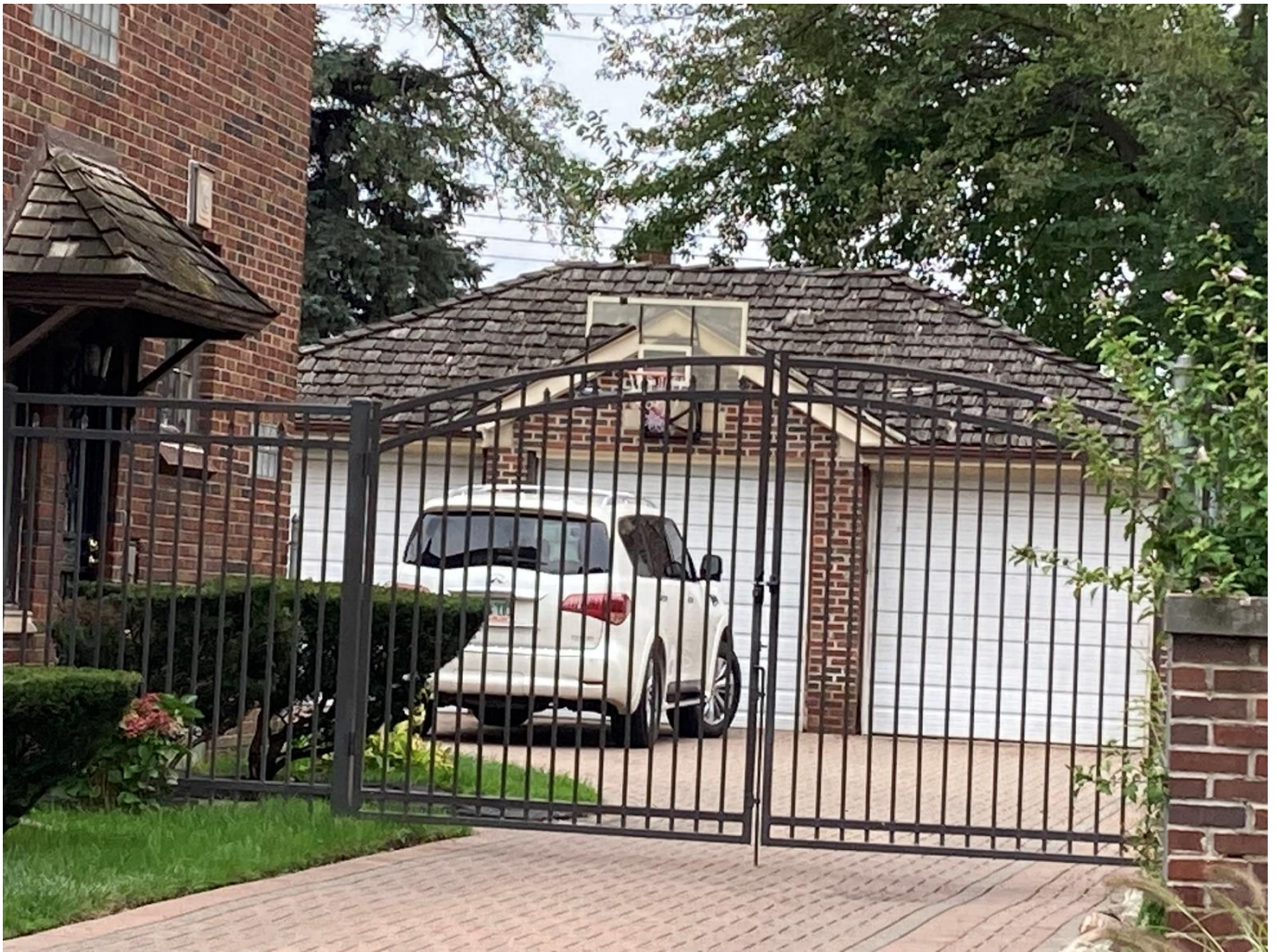
19219 Warrington Drive, garage's front (east) façade, September 2025, staff photo.
