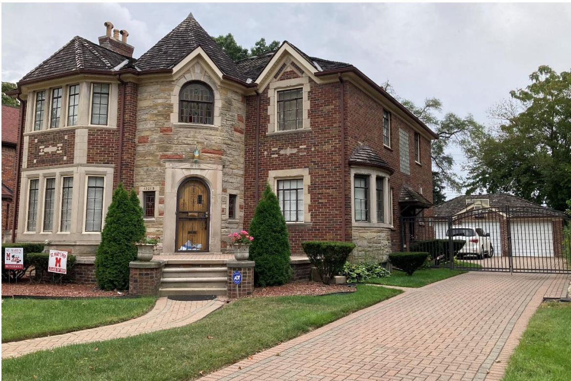
19219 Warrington Drive, front (east) façade, north side, and garage, September 2025, staff photo. Wood shingle roof evident on both house and garage.
