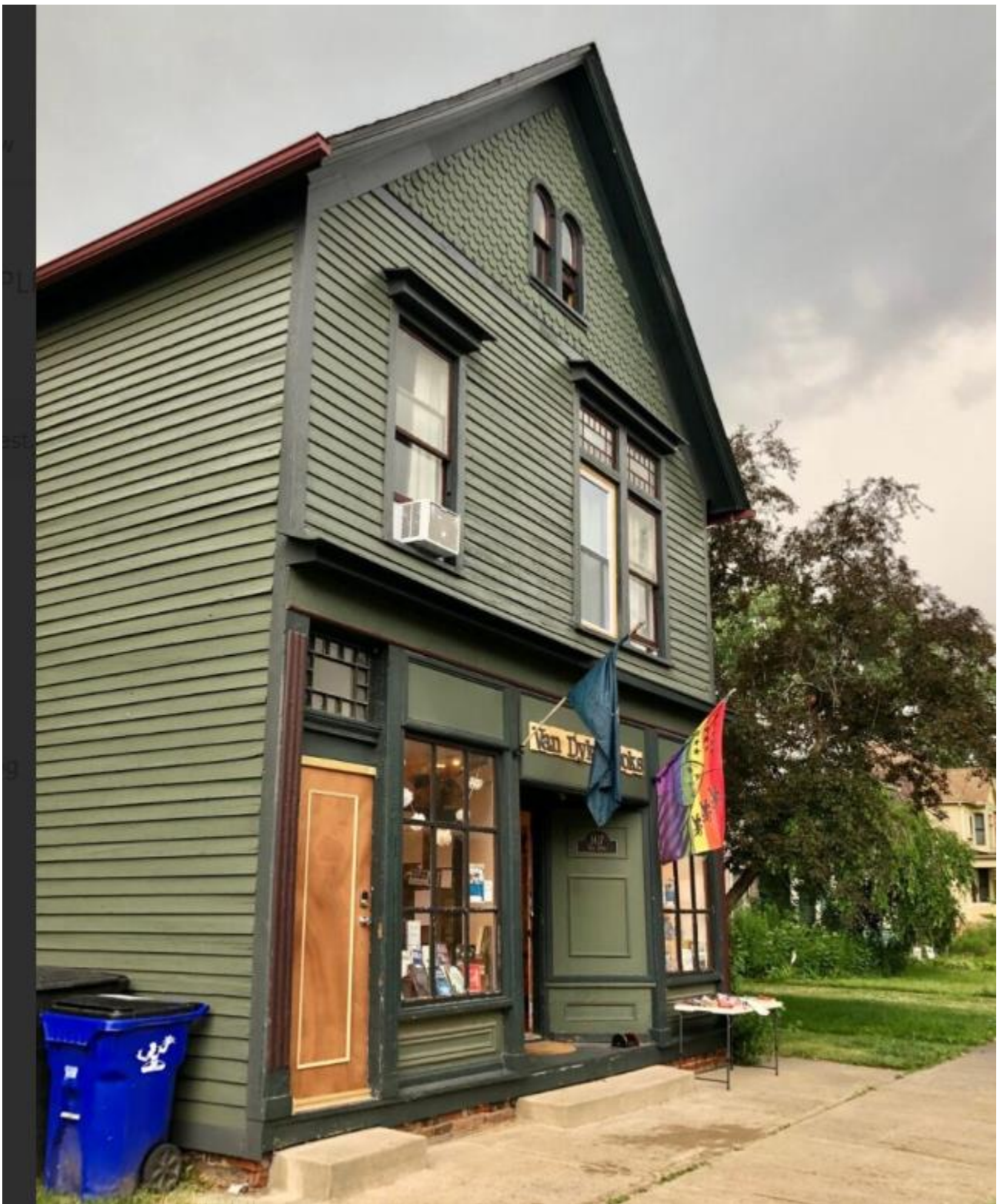
1417 Van Dyke (AFTER), 2024 by HDC staff. Note original lapped wood siding is now revealed and restored
