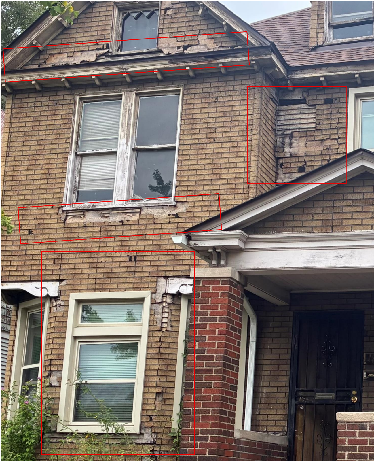
Front façade. Areas outlined in red show deteriorated faux brick/asphalt siding Photo taken on 9/22/2025 by HDC staff
