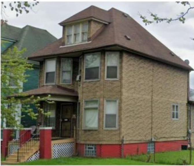
1773 Parker, Google Streetview 2019 (left), with faux brick/asphalt siding (BEFORE). Photo at right taken by HDC staff in 2024, showing original/repaired lapped wood siding (AFTER)
