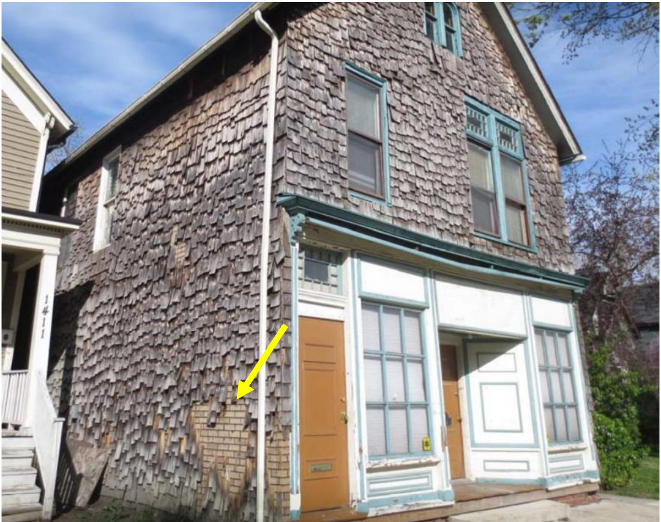
1417 Van Dyke (BEFORE), Google Streetview 2013. Note the presence of faux brick/asphalt siding (yellow arrow) underneath wood shake.
