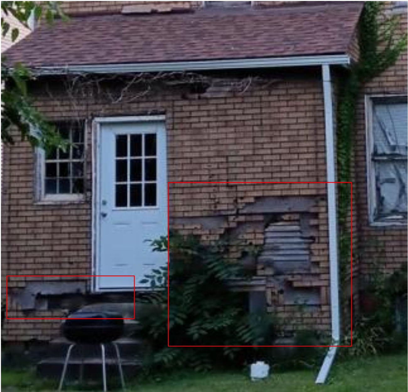
Rear façade. Areas outlined in red show deteriorated faux brick/asphalt siding Photo taken applicant.
