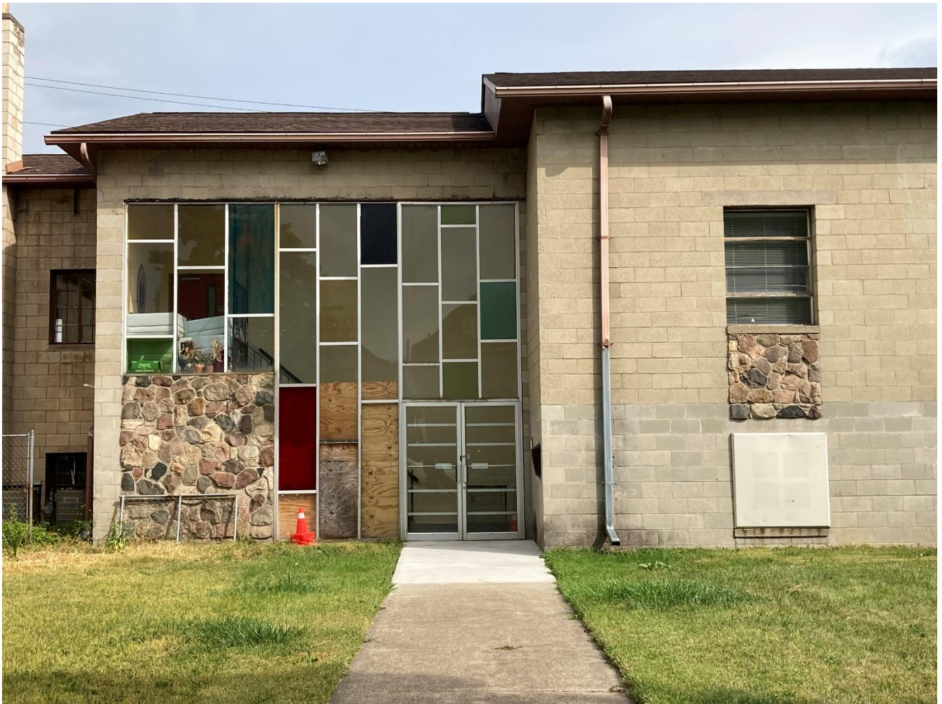
Detail, 1963 glassed-in vestibule. Window wall with aluminum doors shown and the rest of the 1963 addition is to the right of the image. The 1963 window wall, entry doors, and windows shown here are all proposed for replacement. (Staff photo, September 2025.)
