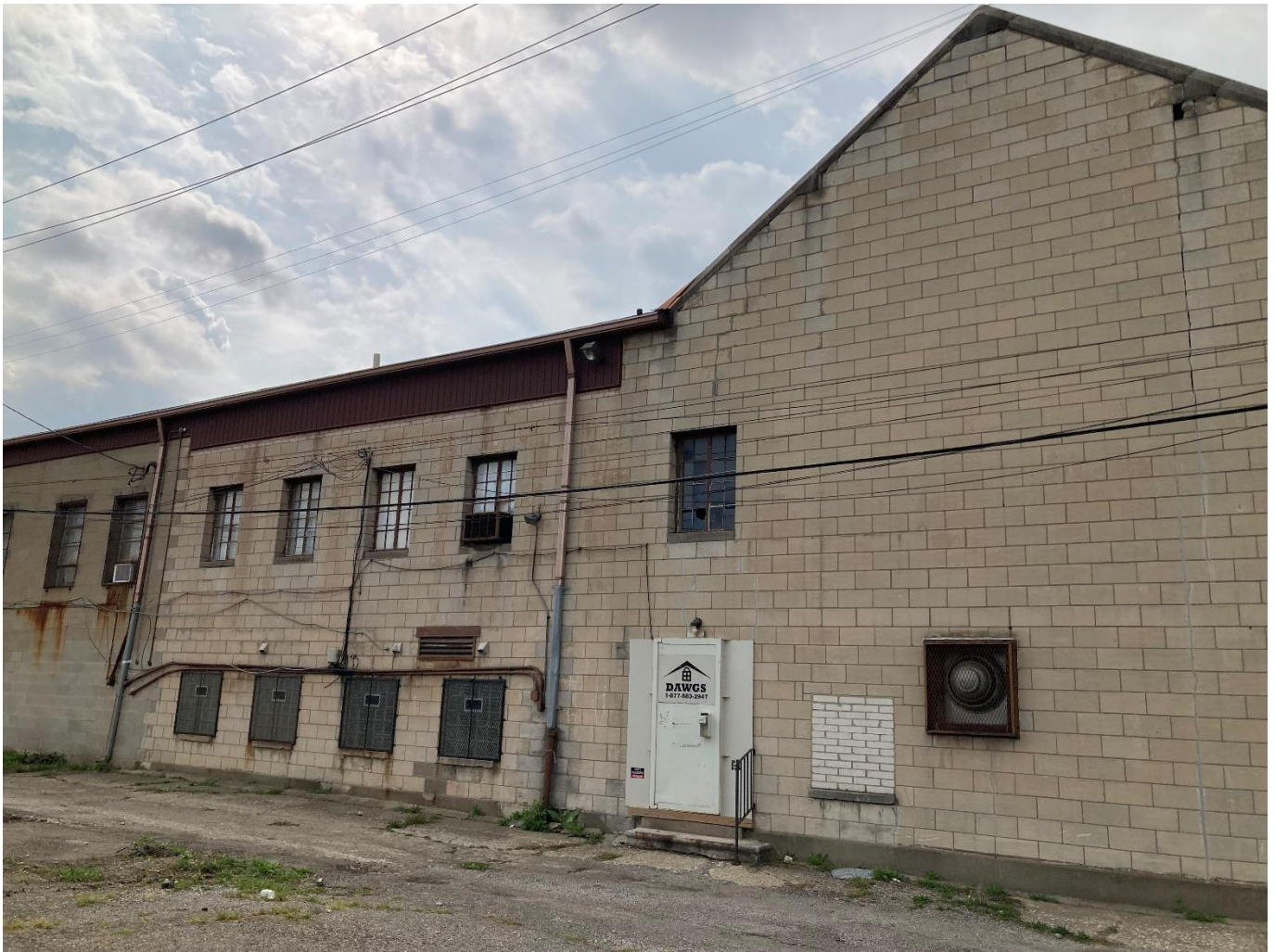
East wall of the 1938 portion and some of the 1963 portion just visible, staff photo, September 2025. Masonry cracking is more visible here. The basement windows shown here will remain in place, All other windows pictured here are proposed for replacement. The 1963 windows are referred to as W1s on the architect's drawings, and the 1938 casement windows here are W4s.
