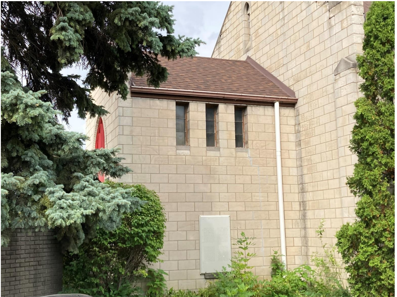
The south side of the 1938 entry hall with three steel windows. These windows are mirrored on the north side of the entry hall and are referred to as W7s on the architect's drawings. These windows are proposed for replacement. This covered basement window is not mentioned in the application materials. (Staff photo, September 2025.)
