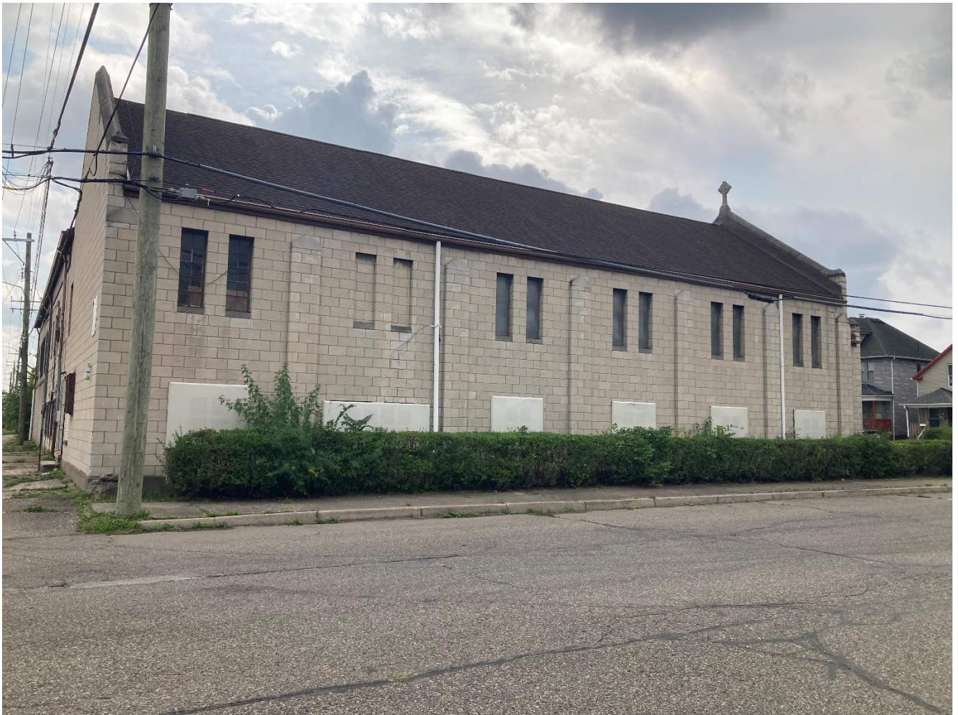
North side of the church, along Milford Street, staff photo, September 2025. Sanctuary windows and covered basement windows are visible. The covered basement windows in this photo are proposed for replacement and are labeled Window 5s and 8s on the architect's drawings. The 8 sanctuary windows will remain in place, but the two narrow windows closest to the northeast corner are 2 W11s on the architectural drawings and they are to be replaced.
