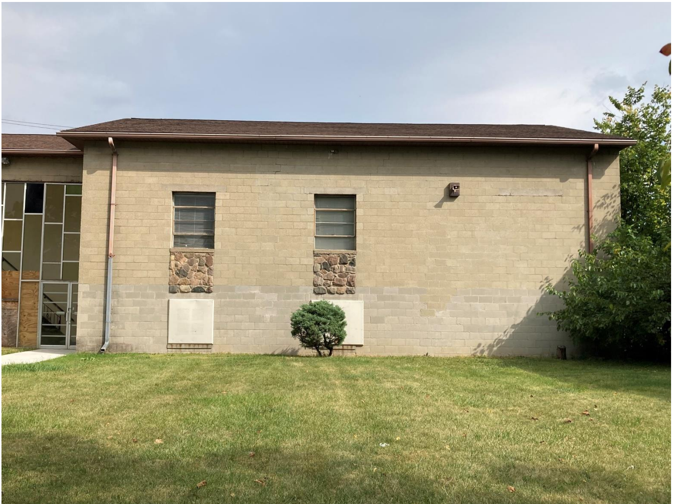
Complete block portion of the west wall of the 1963 addition shown, September 2025, staff photo. All four windows on the block portion of the building (two W2s and two W9s) are proposed for replacement.
