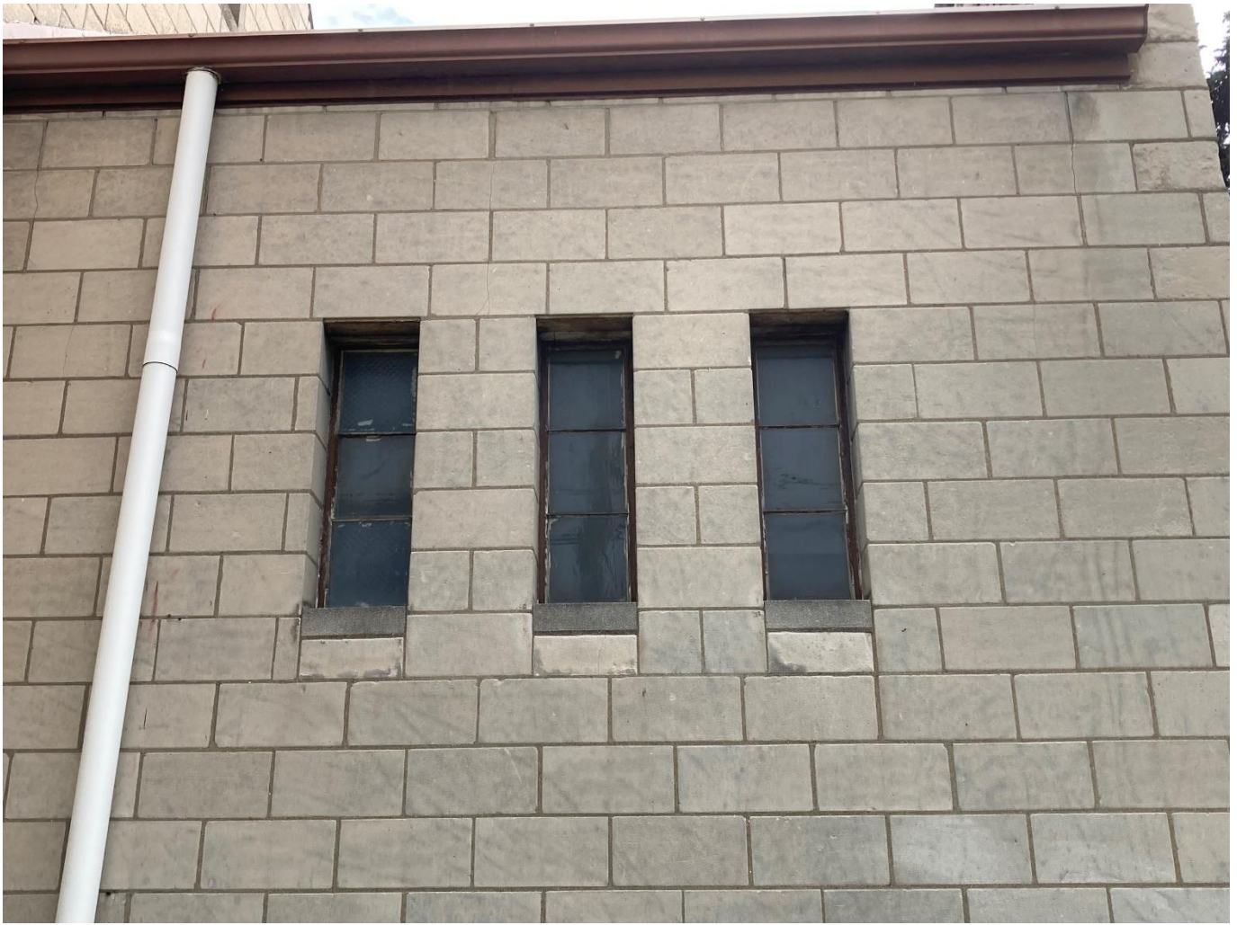
Detail of the three north-side windows on the 1938 entry hall. Windows are steel with narrow muntins. Staff photo, September 2025.
