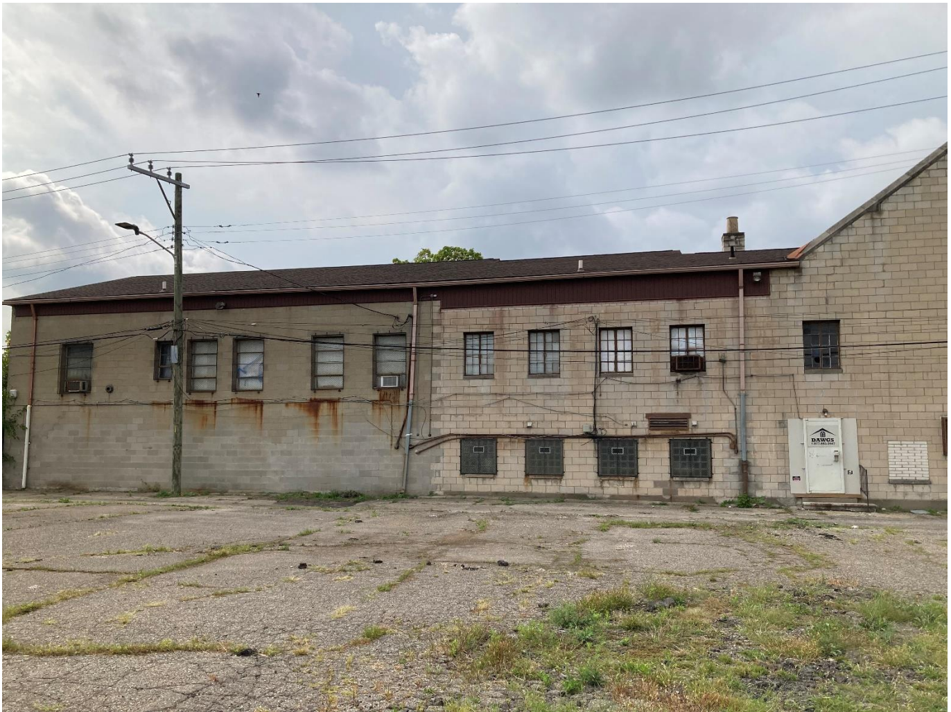
East wall from parking lot behind church, staff photo, September 2025. 1963 portion to the left and the 1938 portion on the right. The 1963 windows with the three horizontal muntins (Window types W1, 2 and 3 on the architect's drawings) and the 1938 steel windows with the narrow horizontal and vertical muntins (Window W4s) are both visible. The basement windows have been infilled with glass block and covered with metal security screens. The basement windows shown will remain, and all other windows shown in this photo are proposed for replacement.
