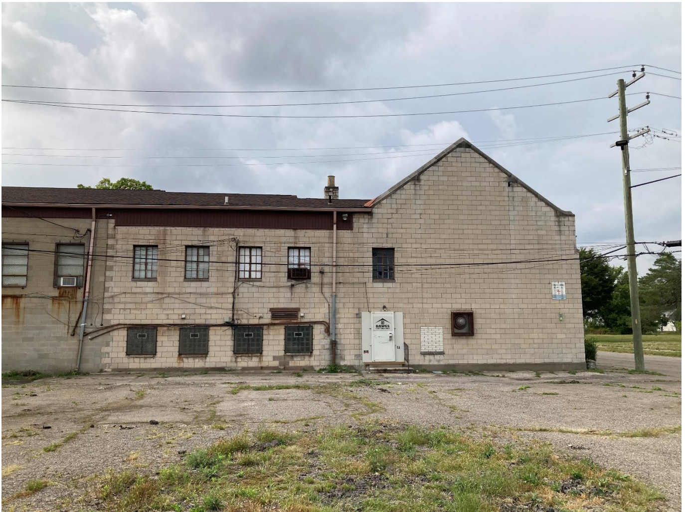
East wall of 1938 portion/ east end wall of the sanctuary. A modern door, bricked-in opening, nonhistoric fan, and steel windows are visible. Some cracking in the masonry near the gable is also visible, perhaps caused by a water drainage issue. Historic steel windows are visible, basement windows with glass block are also visible, and the joint with the 1963 portion can be seen to the left. The four basement windows here that have been infilled with glass block will remain in place. All other windows shown here are proposed for replacement and are labeled Window W1s on the 1963 portion and W4s on the 1938 portion on the architectural drawings with this application. (Staff photo, September 2025.)
