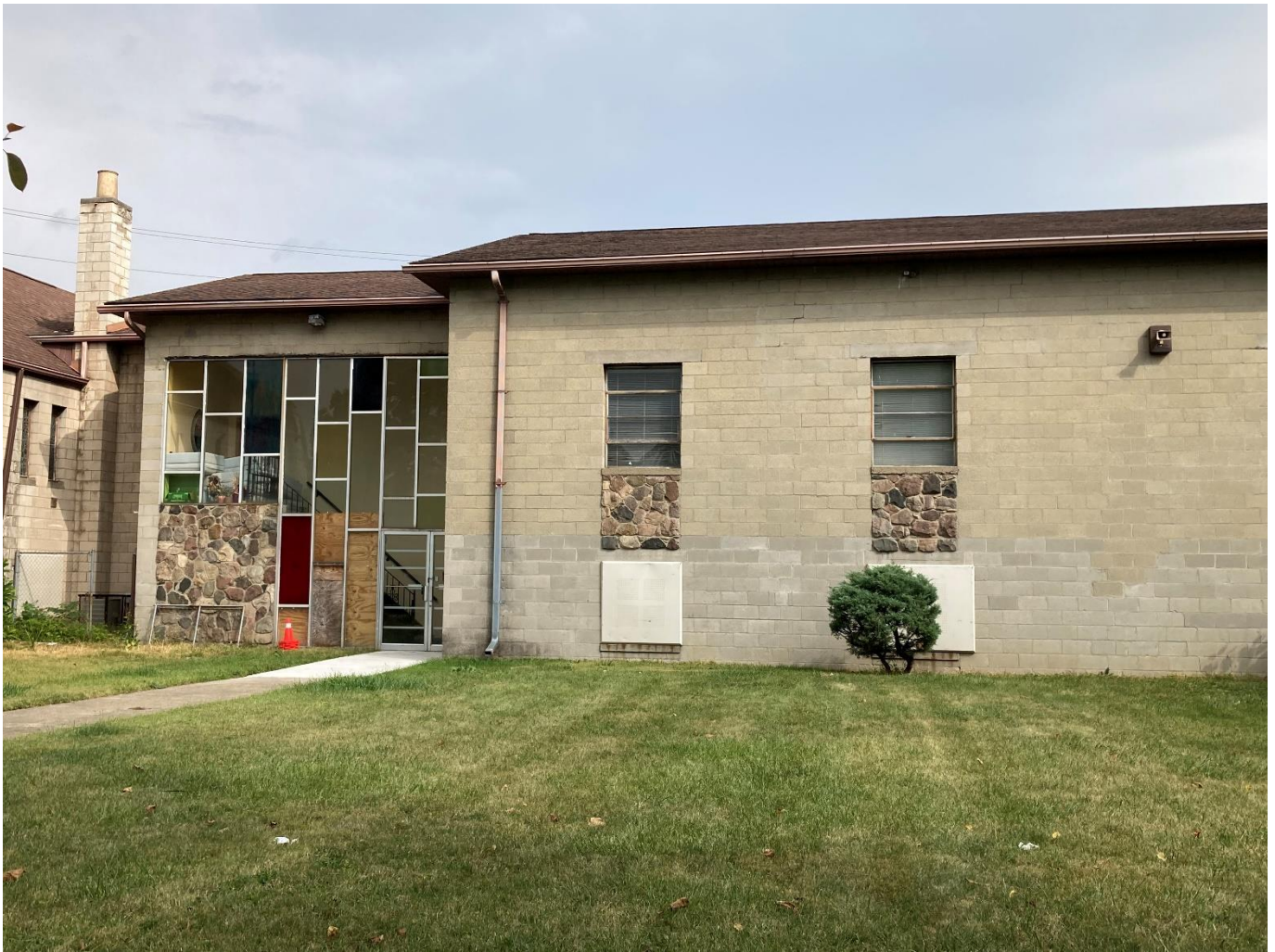
Most of the west façade of the 1963 addition shown, staff photo, September 2025. The stone veneer panels on the glassed-in vestibule and below the windows are visible. The glassed-in vestibule and the four windows shown in this photo on the 1963 addition are all proposed for replacement. The windows with the stone below are labeled W2s on the architect's drawings, and these basement windows are labeled W9s.
