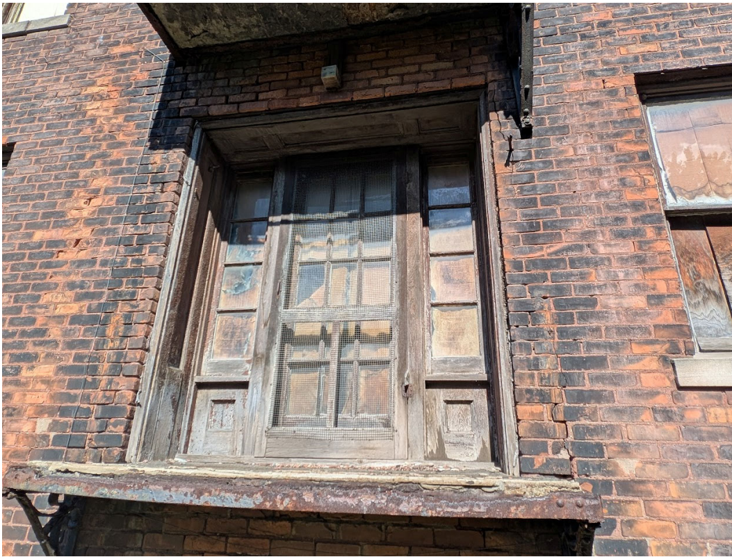
Detail view of west side “balcony” historic-age entrance system, a single 15-lite in-swing door flanked by 3-lite sidelites. Staff photo. These units are proposed for replacement by the applicant. August 28, 2025.
