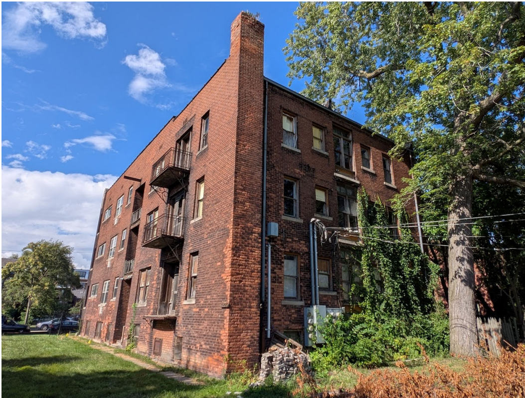
View of 467 West Alexandrine, rear quarter view looking back towards street. Note advanced deterioration of common brick in this area. Staff photo, August 28, 2025.
