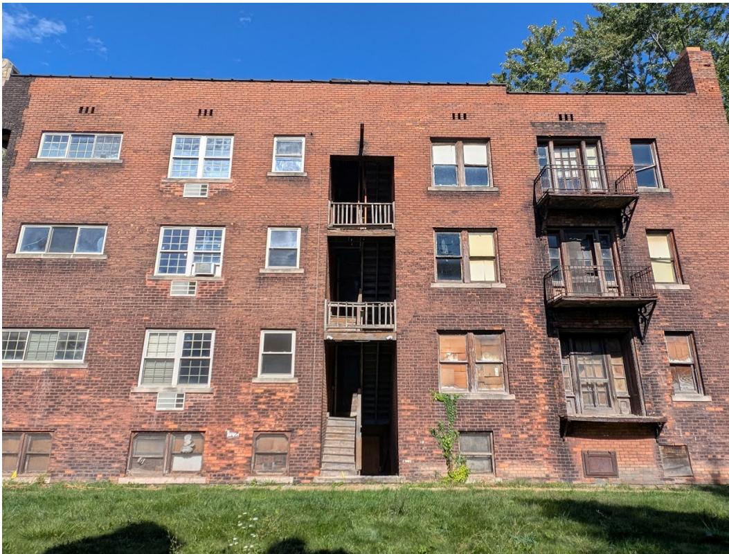
View of 467 West Alexandrine, to the east, showing west-facing side. Note wooden windows/doors on right side (towards building rear). The ornamental face brick (brown) at front of building, wrapping around, is just visible in upper left of photo, distinguishing it from the common brick at this utilitarian side. Staff photo, August 28, 2025.
