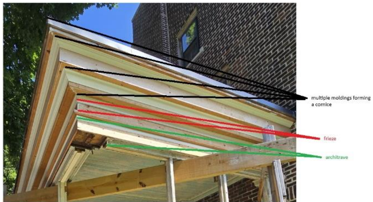
Comparing the front historic feature (top) with the newly built feature on the west porch (bottom), using photos from the applicant's materials. The historic cornice projects out over the frieze and architrave. It seems that the modern construction stacks trim to progress from the frieze to the roof.
