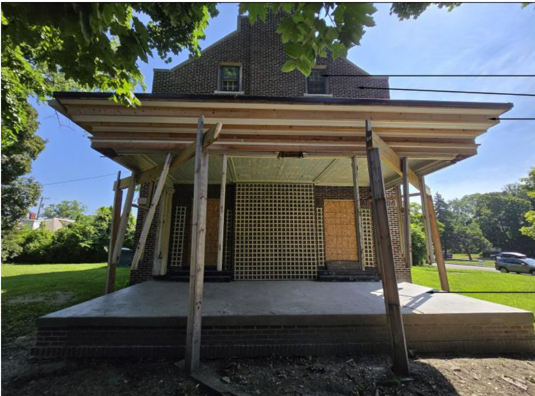
Applicant Photo, west elevation. Columns are missing. New brick base, concrete cap, and entablature has been built.
