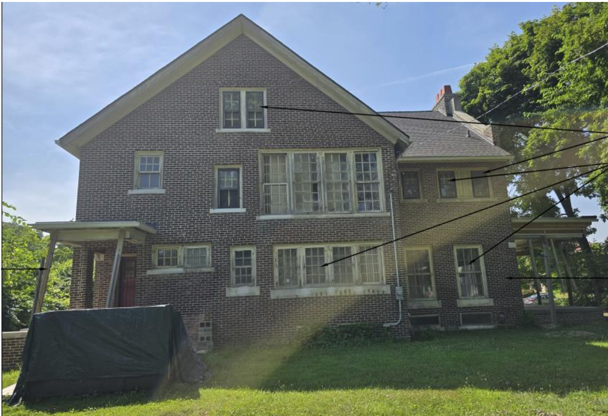
Applicant Photo, rear (north) elevation, current conditions. Rear porch columns are missing.
