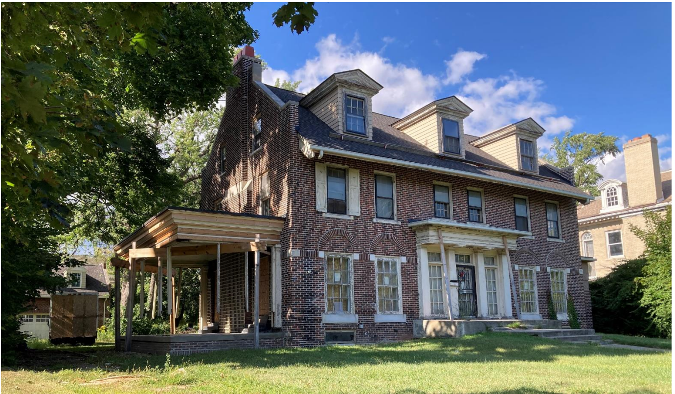
Site Visit, Photo 2, staff, August 2025. West porch columns have been removed and porch entablature has been rebuilt but also somewhat reinterpreted. See detail photo on page 4.
