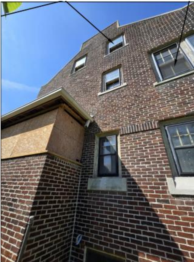
Applicant Photos, east elevation, missing windows behind the boards.
