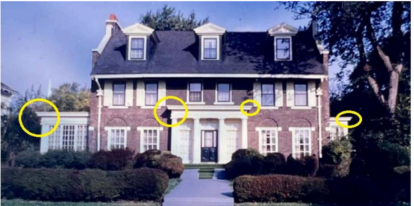
1981 designation photo with entablatures circled. The same classical entablature above the classical column both on the west and on the front portico is important to this house's design, character, proportions, and balance.
