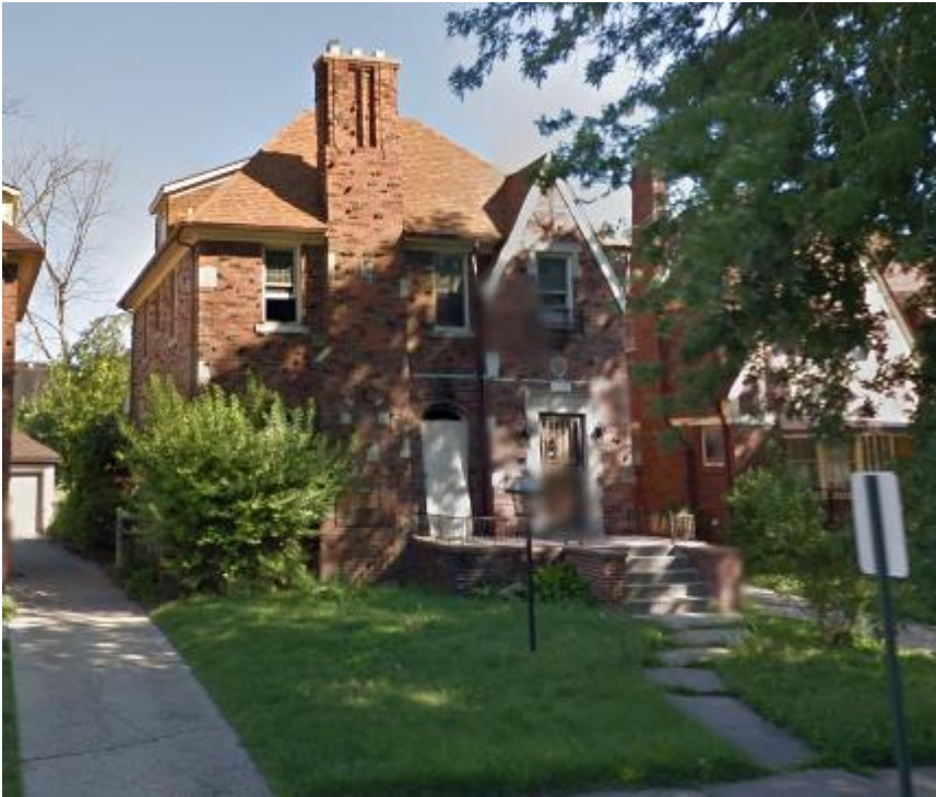
Google streetview, August 2011. Second-floor windows appear open and a board is leaning against the first-floor window, but the decorative railing below the second-floor window, the low decorative railing around the front porch, and the storm door are all intact. Shrub is overgrown.
