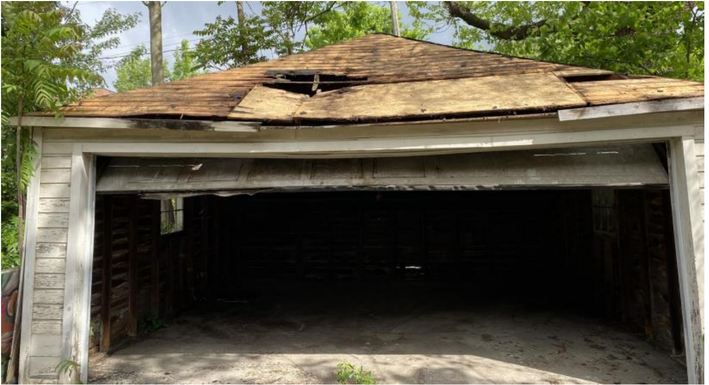
Applicant-provided photo from application of garage in current condition. Applicant states that the plan is to replace roof and repair and repaint wood siding, replacing in kind as needed. The garage door is not mentioned.
