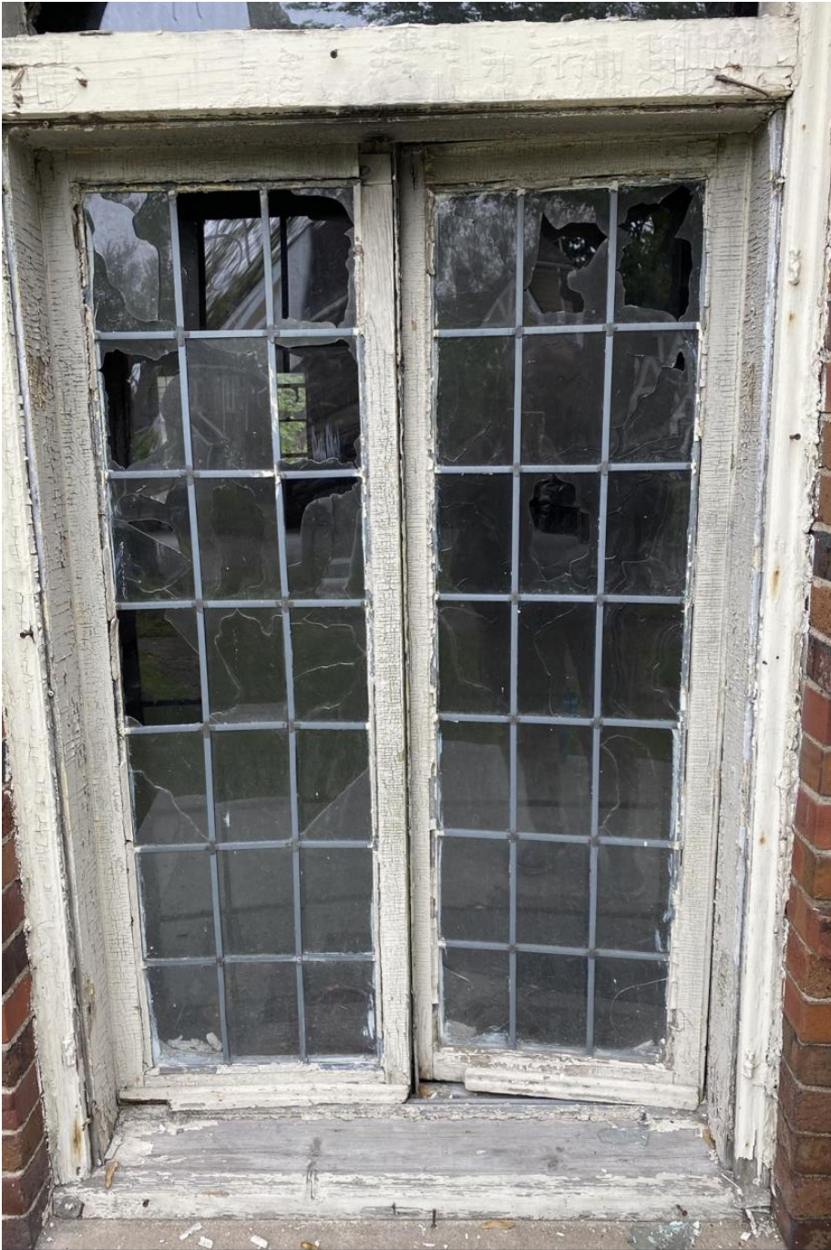
Applicant's photo from their initial application. First-floor casement windows with leaded glass on the front façade. Cracked paint and some broken glass are visible.
