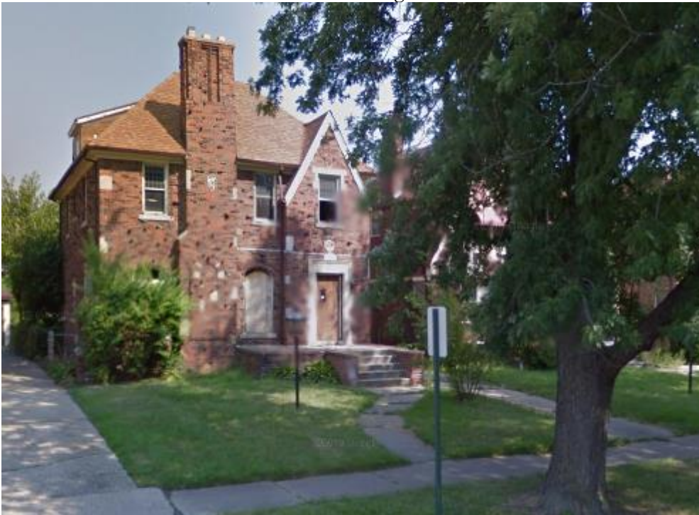
Google streetview, August 2013. Second-floor windows are in the same position as in 2011. First-floor window is covered or boarded. Exterior storm door, second-floor decorative railing, and low porch railing are all gone. Shrub is overgrown.
