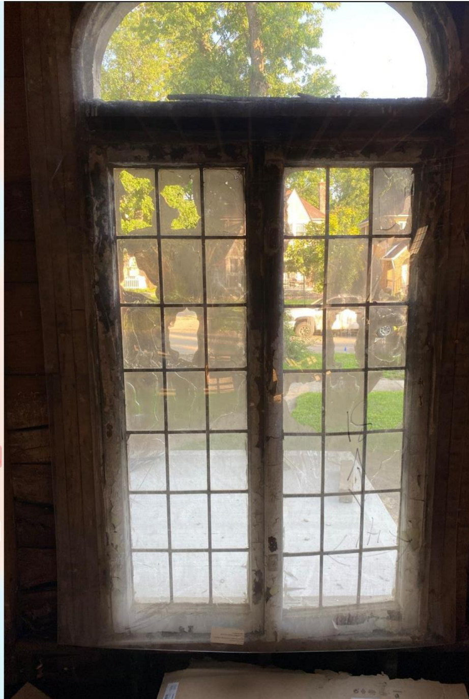
Applicant's photo from updated application materials. One of the first-floor casement windows from the interior. Some broken panes of glass and some deteriorated paint are visible.
