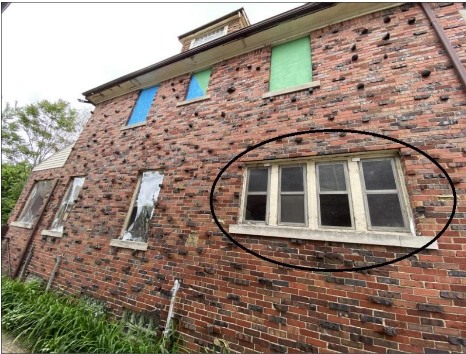
Applicant's photo from updated application materials, west elevation. Some windows are boarded, some may be missing, but these circled windows with mullions between may be present. Their conditions are not described in the applicant's materials.
