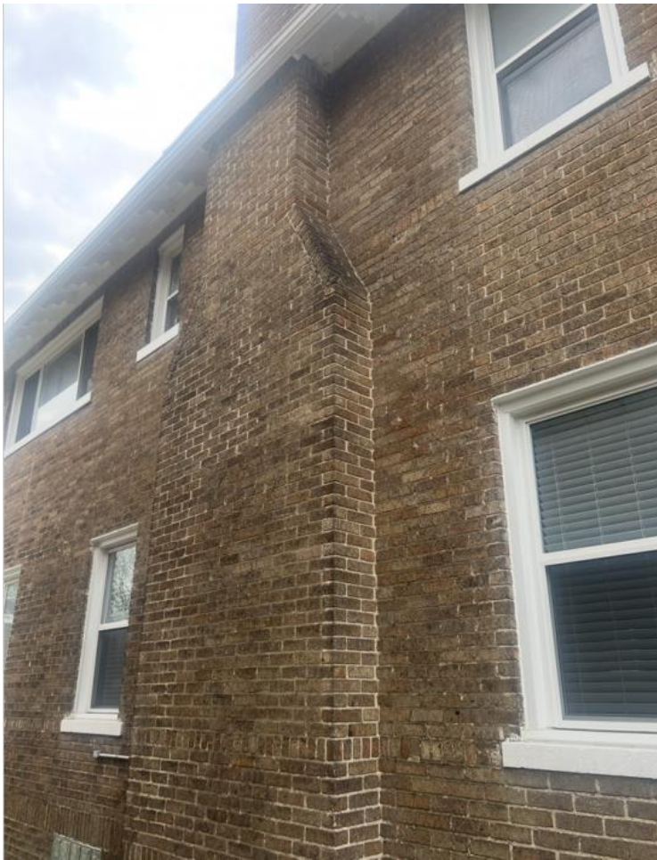
East side wall. Note incompatible vinyl 1/1 and slider units with aluminum trim/brickmould. Photo by HDC staff, 2024
