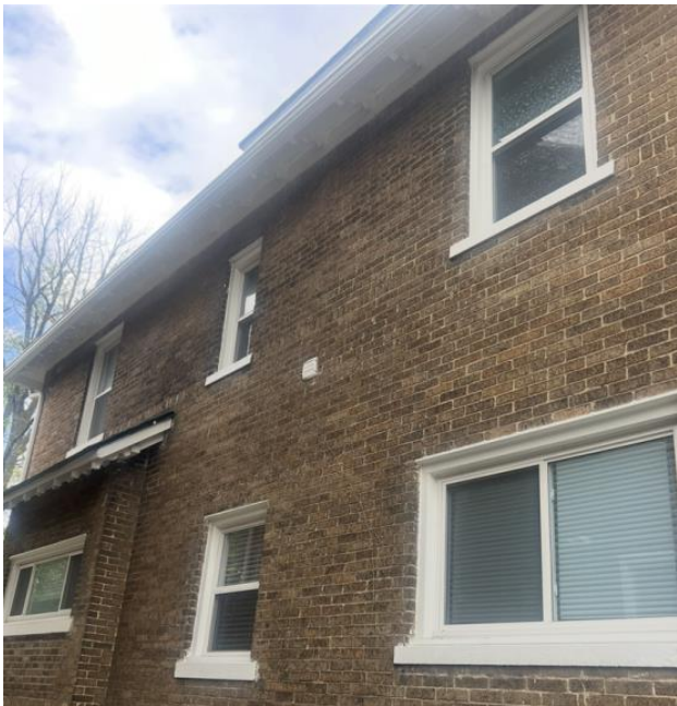
West side wall. Note incompatible vinyl 1/1 and slider units with aluminum trim/brickmould. Photo by HDC staff, 2024
