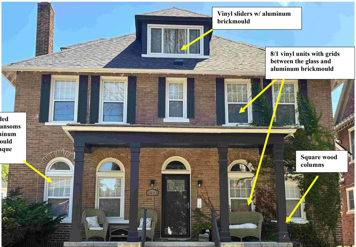
Current condition. Photo by HDC staff, 8/26/2025. Note unsympathetic alterations which have removed elements associated with the building's Colonial Revival style
