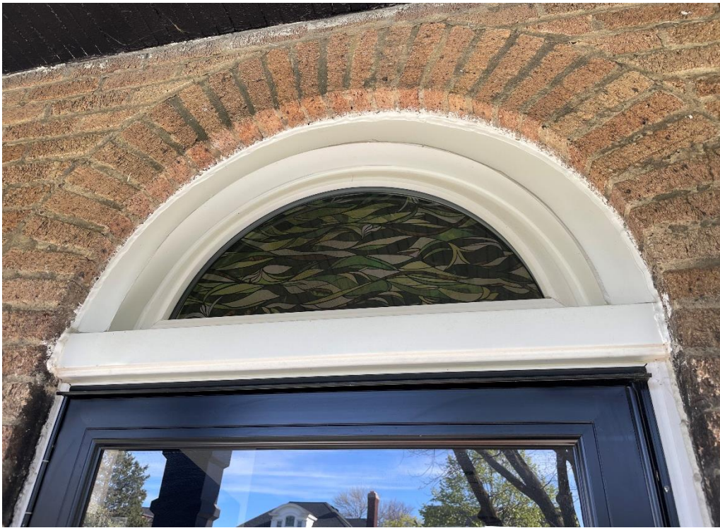
Current condition. Photo by HDC staff, 2024. Detail of incompatible opaque glass, vinyl windows, and aluminum brickmould at front the front façade, first story
