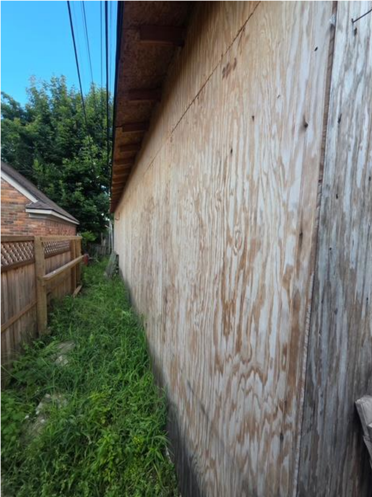
Applicant-provided photo, completed garage, 2025, rear (west) elevation. Unfinished plywood surface visible..
