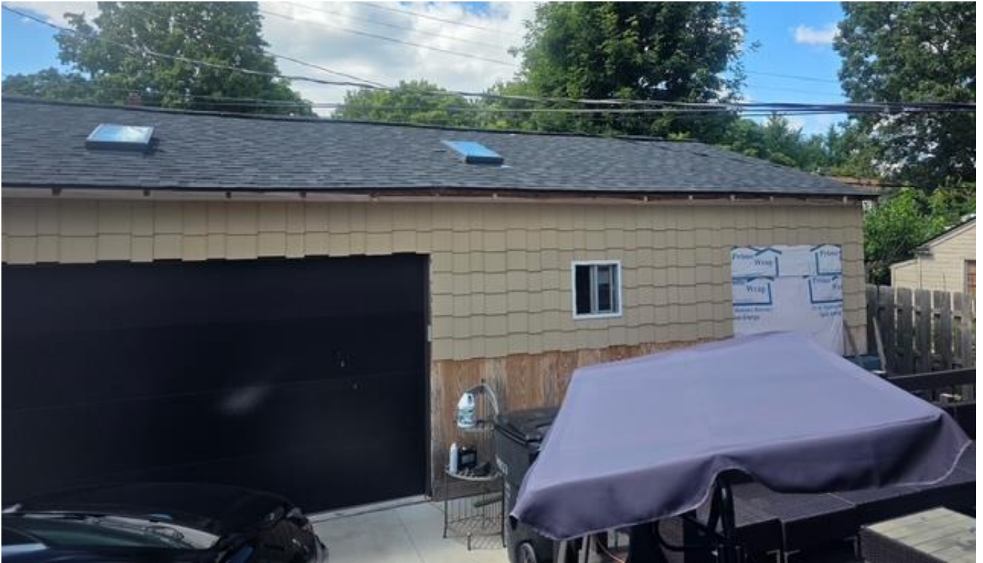
Applicant-provided photo, completed garage, 2025, east elevation. The composite siding, installed garage door, installed window, and skylights are visible. Next to the window is the unsided area where the sliding glass door is proposed.
