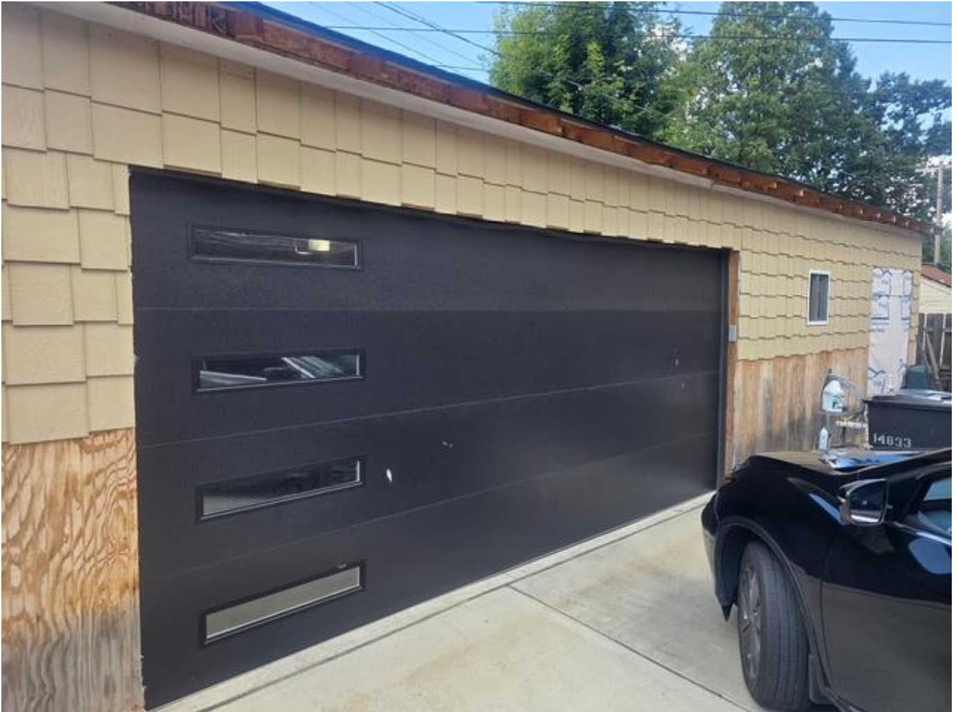
Applicant-provided photo, completed garage, 2025, east elevation. The composite siding, installed garage door, and installed window are visible. Next to the window is the unsided area where the sliding glass door is proposed.
