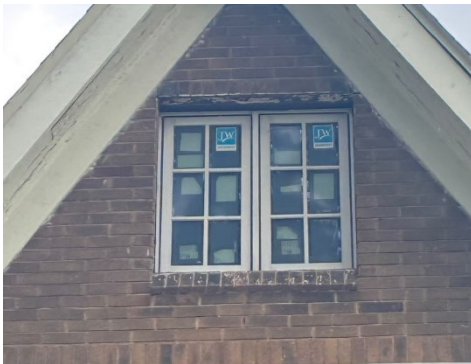
Current aluminum-clad wood replacement windows, brickmould, and mullion.
