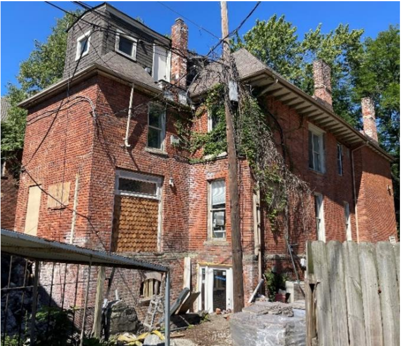
Photo 5. 691 W Canfield, September 2022, staff photo, post unapproved demolition work. The south end of the house still looks much like this in 2025. The south end of the house is shown where a single door and a window opening are boarded up. That door used to step out onto the rubble-and-concrete deck between the house and the retaining wall, and the bricks with white staining below the door and window were not visible because of the former deck. The wide door opening infilled with a transom and fishscale shingles near the house's southeast corner used to be double doors that opened onto the rubble-and-concrete deck. These boarded-up and infilled openings are part of this application. The door with sidelights visible here below grade at the house's southeast corner is the door with sidelights proposed in this application again, but painted a new color. That door would not have been visible either, when the former deck was in place, but the demolition exposed this area and the proposed new deck will not cover this area up. In the applicant's proposal, the door with sidelights would remain exposed and would open to a sunken patio.
