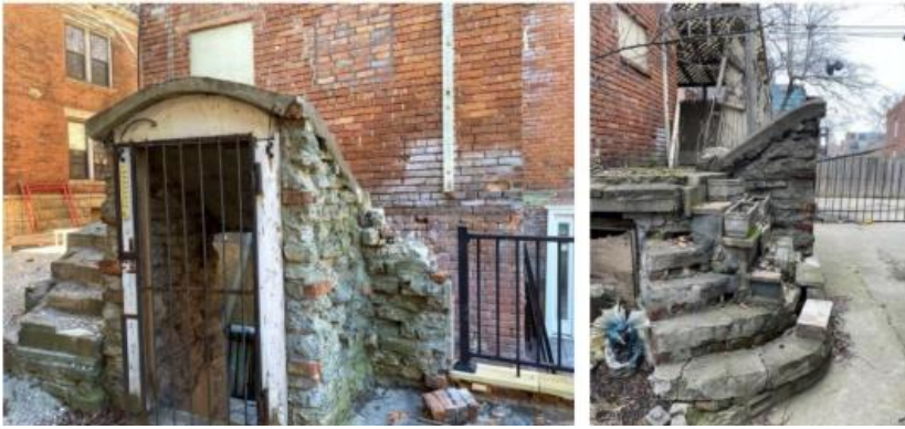
Photo 6. Photos of the house's south end provided by applicant's consultant in a report that has been included in the application. All of the stone and concrete construction visible here, along with the wood porch/pergola construction further east, are "proposed for demolition." In reality, much of that material has been demolished and only the rubble-and-concrete vault-like structure remains; it, too, is proposed for demolition.
