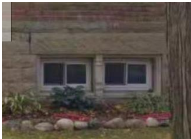
Photo 7. 691 W Canfield, front (north) elevation, basement windows visible below the large stone arch and picture window with transom toward the east side of this elevation, October 2020, Google streetview. The carved mullion between the two windows was visible in 2020 and is proposed to be replicated in 2025.
