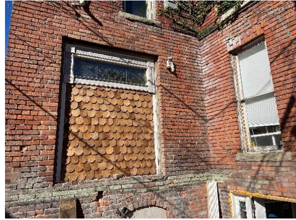
Site Photo 11 by staff, September 1, 2022 : (South) rear, east-facing elevation showing location of removed French doors and infill with fish-scale siding and stained glass transom from another building installed in the opening.
