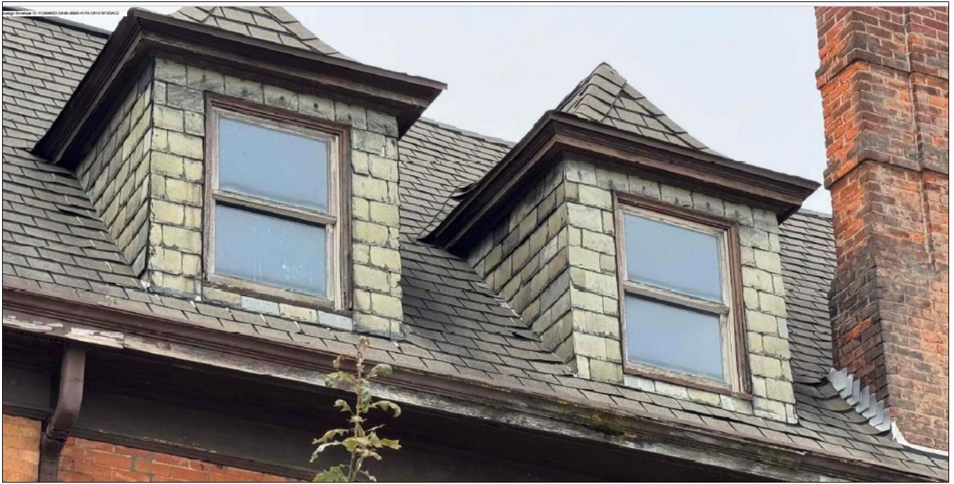
Photo of slate tiles on east dormer walls, prior to removal, from application HDC2025-00701.
