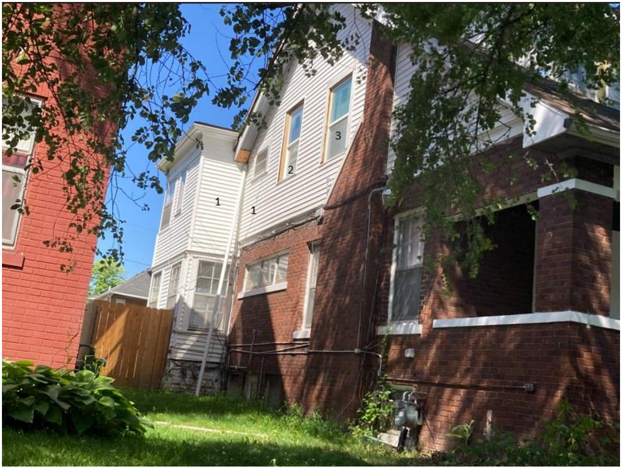
Figure 3. Staff marked up Photo 3 of the house's south side from June 2025 to show the new elements staff can see plainly from the sidewalk, marked with red triangles. Those recent changes include the two new windows where six-over-ones used to be, and the white vinyl siding installed over the historic gray wood siding on the house. It is currently unknown what material covered the rear addition before the white vinyl. The addition on the north side had gray siding, so it's possible that this part of the addition had gray siding also.
