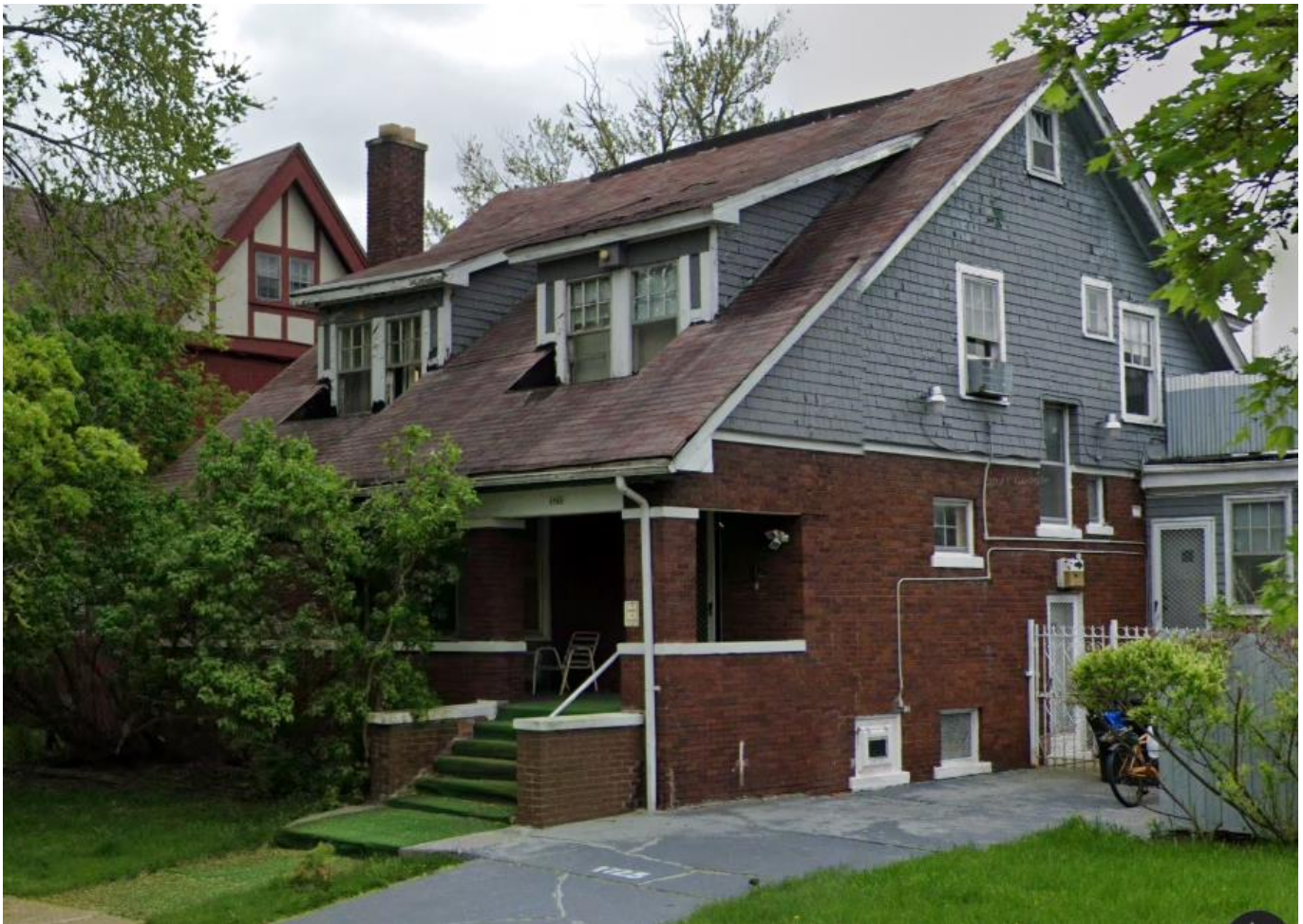
Photo 8, 1725 Seyburn, May 2019, Google streetview, more detailed view. Conditions prior to the recent unapproved work. Note wood windows and wood shake siding at gable ends and dormers.
