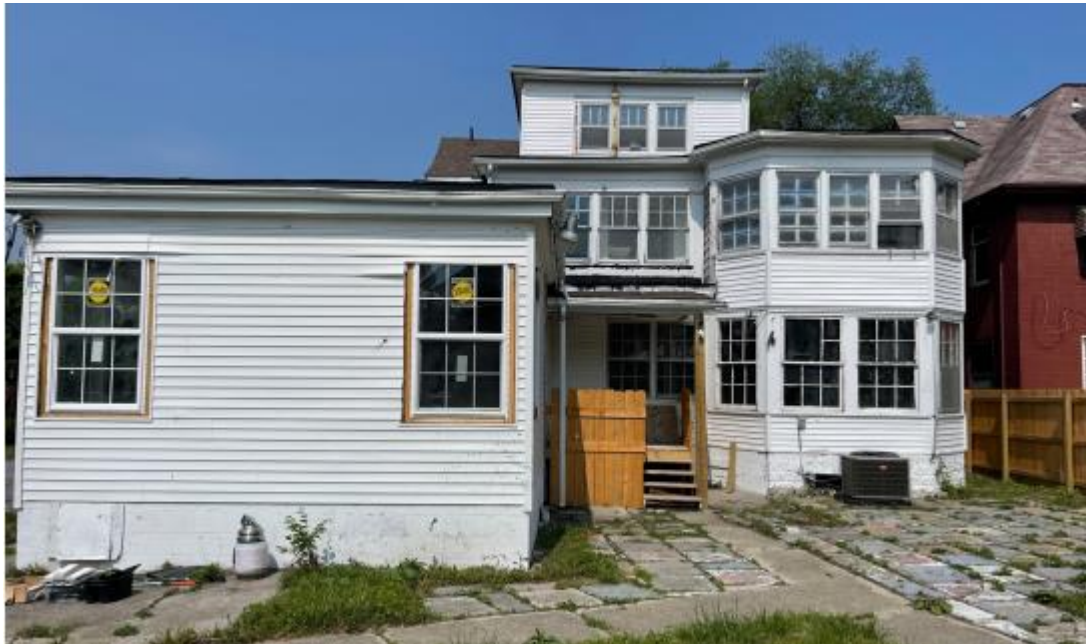
Photo 5, provided by applicant. 1725 Seyburn, rear (west) end, currently sided with white vinyl siding and exhibiting a variety of window types, materials, and configurations. The vinyl siding and the two replacement windows visible here on the one-story addition are included in this application.
