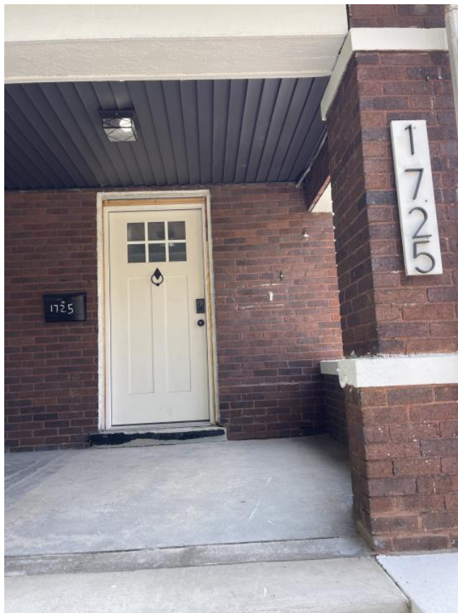
Photo 10, provided by applicant. Photo appears to show lap siding installed on the ceiling of the front porch. Also pictured is the replacement front door and new address plate installed on the brick column.
