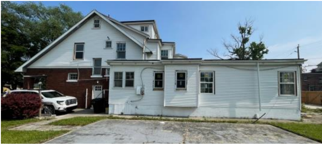
Photo 4, provided by applicant. 1725 Seyburn, north side, original historic house volume and one-story addition toward the northwest corner of the house, currently sided with white vinyl siding and exhibiting a variety of window types, materials, and configurations. The siding and the window replacements are included in this application.
