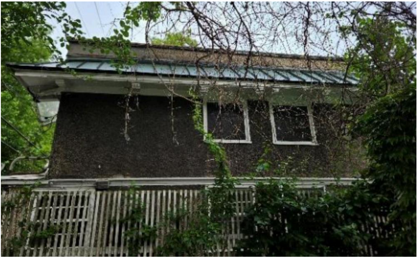
141 W. Boston. Photo provided by applicant. Showing metal roofing at rear garage/carriage house's pent roof/canopy, at the west/side façade. The roof at the east/side façade is also covered with metal roofing
