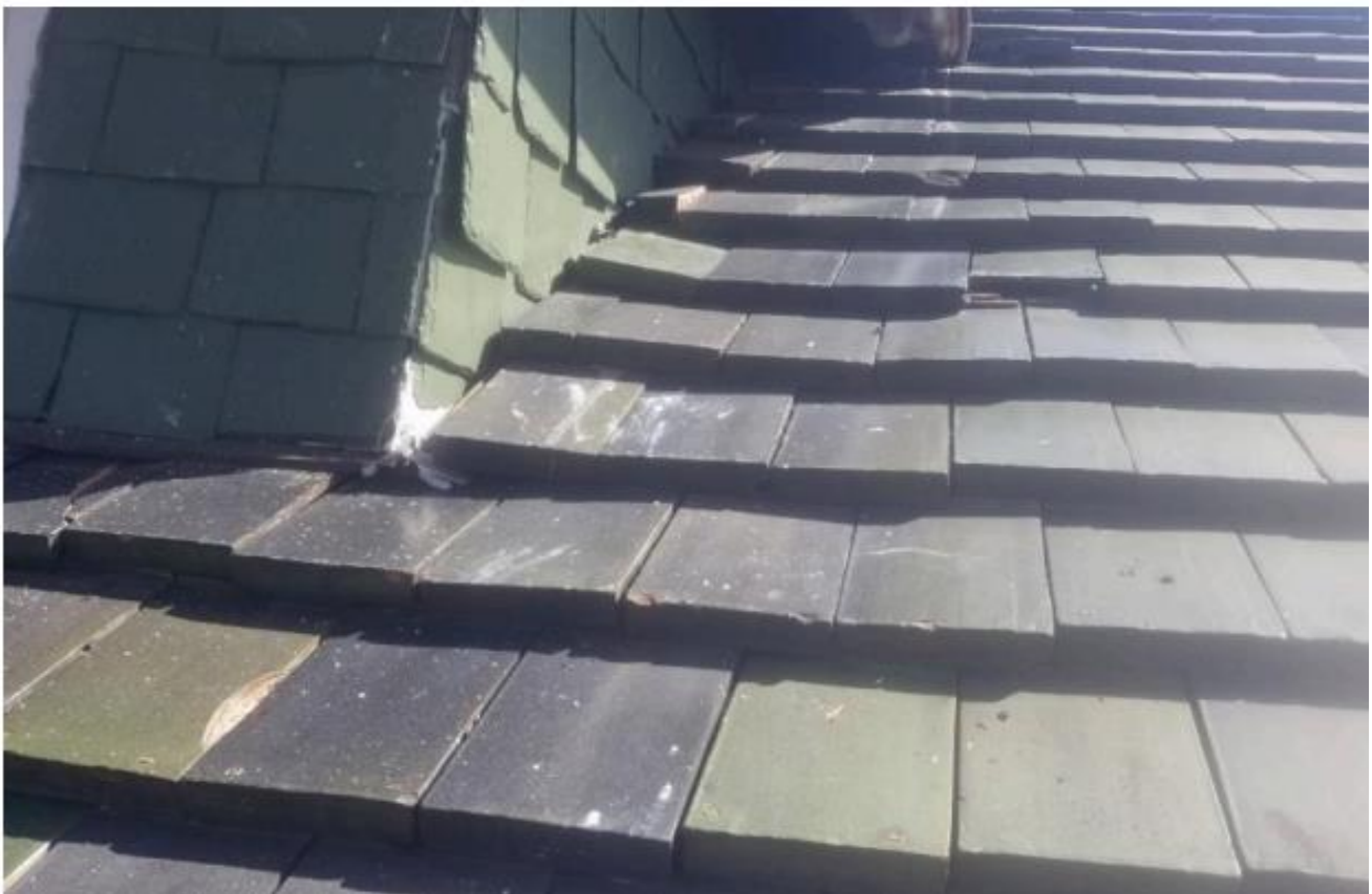
West side dormer, clad with slate, painted green. Photos provided by applicant
