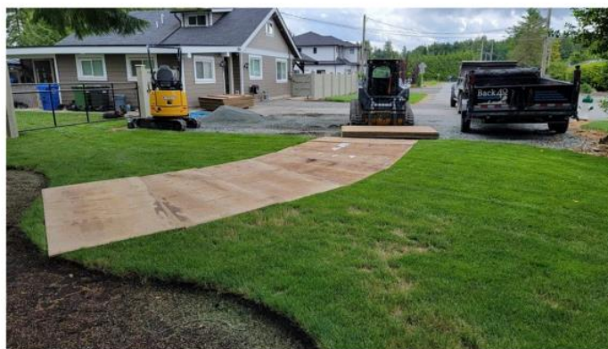
Trunk and limb protection of mature vegetation (left) and \frac{3}{4} " plywood sheets for soil compaction protection (right), from applicant documents (not to scale).
