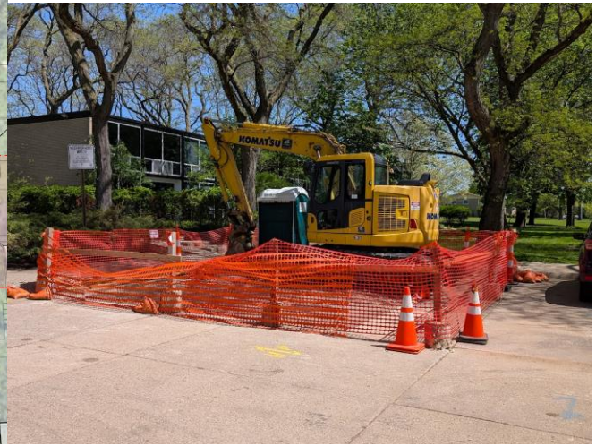
2 – Nicolet Place vicinity, from applicant documents (not to scale). This location will have an open cut zone in the concrete cul-de-sac and will replace manhole lid. The vent stack has been removed from the proposal since the previous submission. Staff photo, May 9, 2025. This work appears to have started but not completed. A small excavator is on site.
