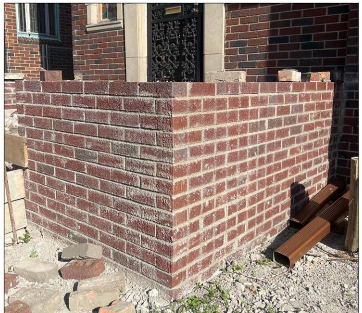
These applicant photos of the rebuilt masonry porch walls were submitted on April 29, 2025 as part of the application for staff review (against which the COA was issued). The bond patterns and mortar joints on both sides of the porch match.
