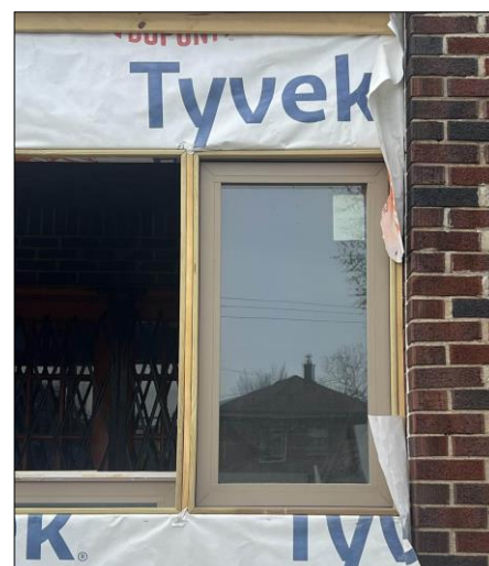
Applicant photo of installed window within newly sized opening.
