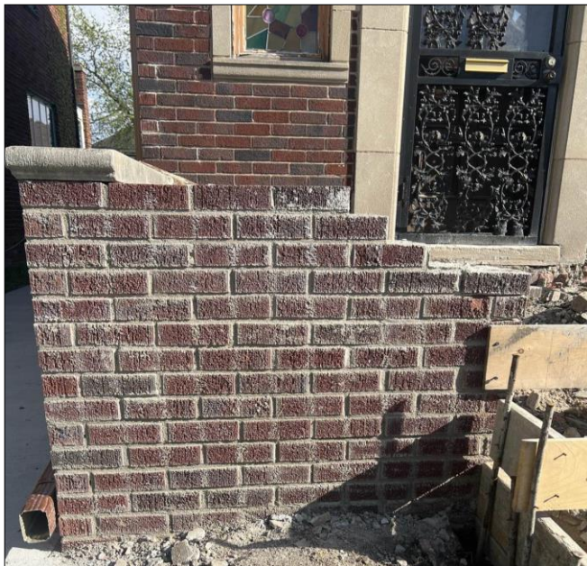
These applicant photos of the rebuilt masonry porch walls were submitted on April 29, 2025 as part of the application for staff review (against which the COA was issued). The bond patterns and mortar joints on both sides of the porch match.
