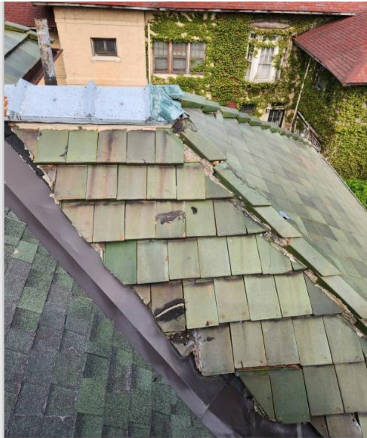
Photo by applicant. Showing area of past roof repair. Note areas of asphalt roofing
