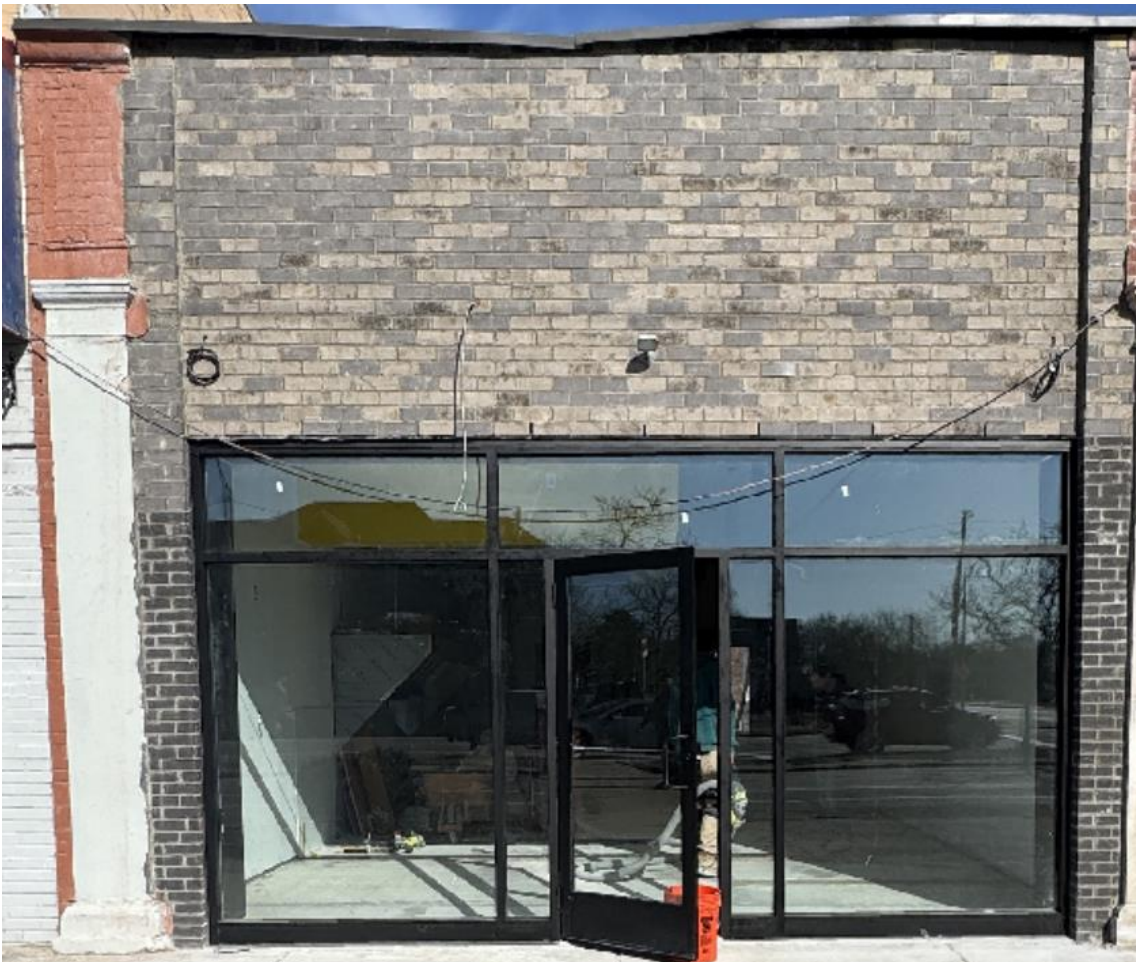
4700 Third Street. Photo from applicant showing current conditions after unapproved brick replacement and storefront installation proposed for approval with the current application (see red arrow). Note all original herringbone pattern at parapet and the limestone band which was below the parapet is no longer present. It appears that the only original portion of the cladding that remains is the limestone pilaster to the left of the new aluminum storefront.
