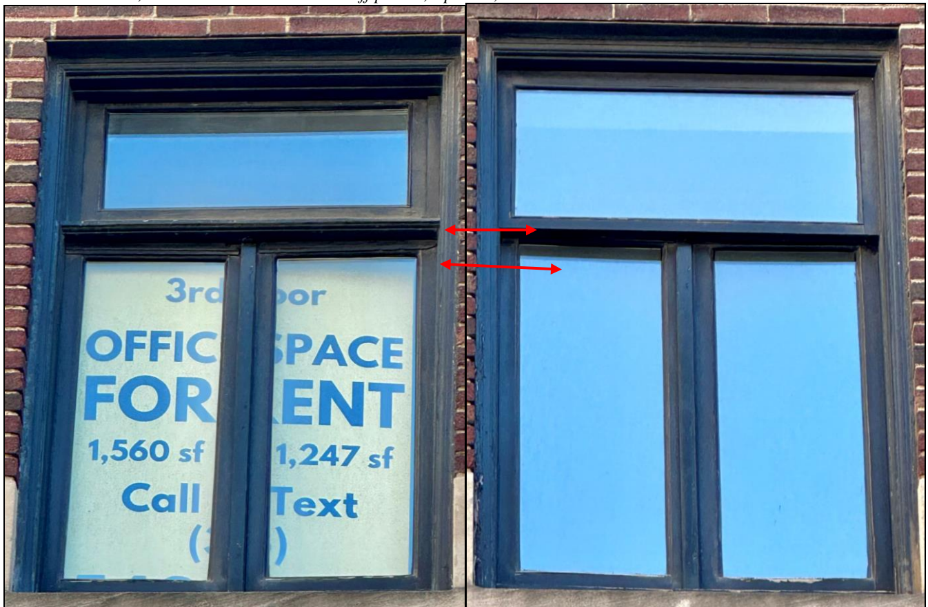
Group A, Second Floor – Both openings have matching highly profiled, and likely original, wood brick mould. The frames of the French windows at left have a visible top sash, whereas the top sash at right is minimally visible.
