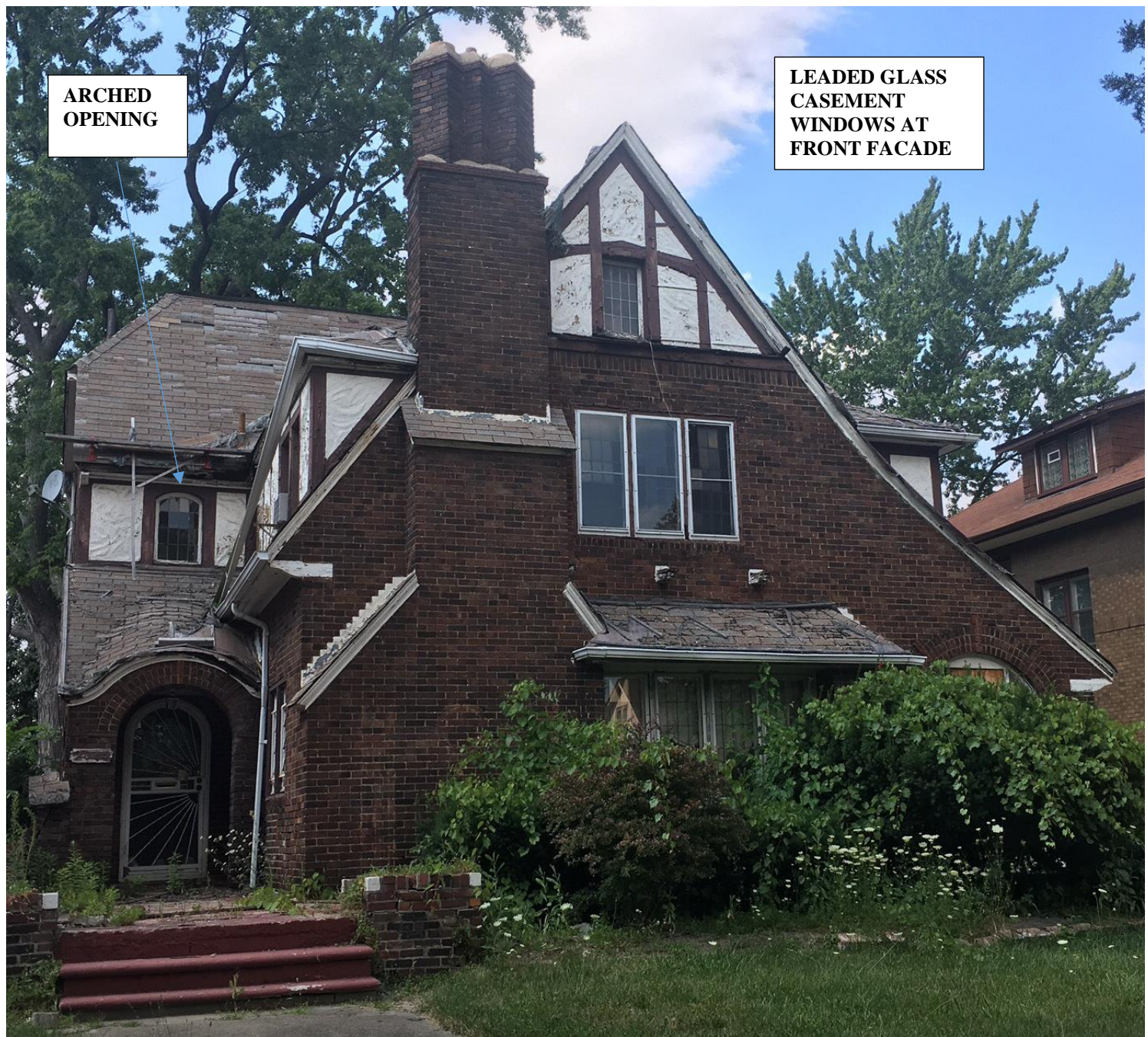
Photo taken in early 2018, prior to the fire. Note that all windows at the front are wood casement windows with leaded glass. The windows at the second story are covered by aluminum windows. Source, HDC files
