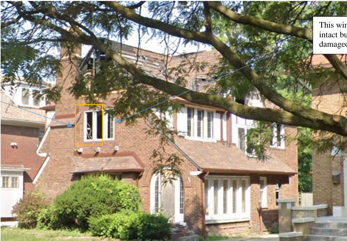
August 2018, after the fire. Note that the windows and associated casing/trim at the side wall and the front door sidelites appear to be intact. Two of the three casement window sash at the front façade, second story (outlined in orange) appear to be completely destroyed although the casing/trim remained. Source, Google Streetview
