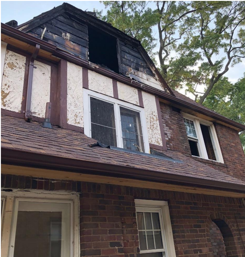
August 2018, after the fire. Detail of fire damage at rooftop dormer, east side. Photo by applicant.
