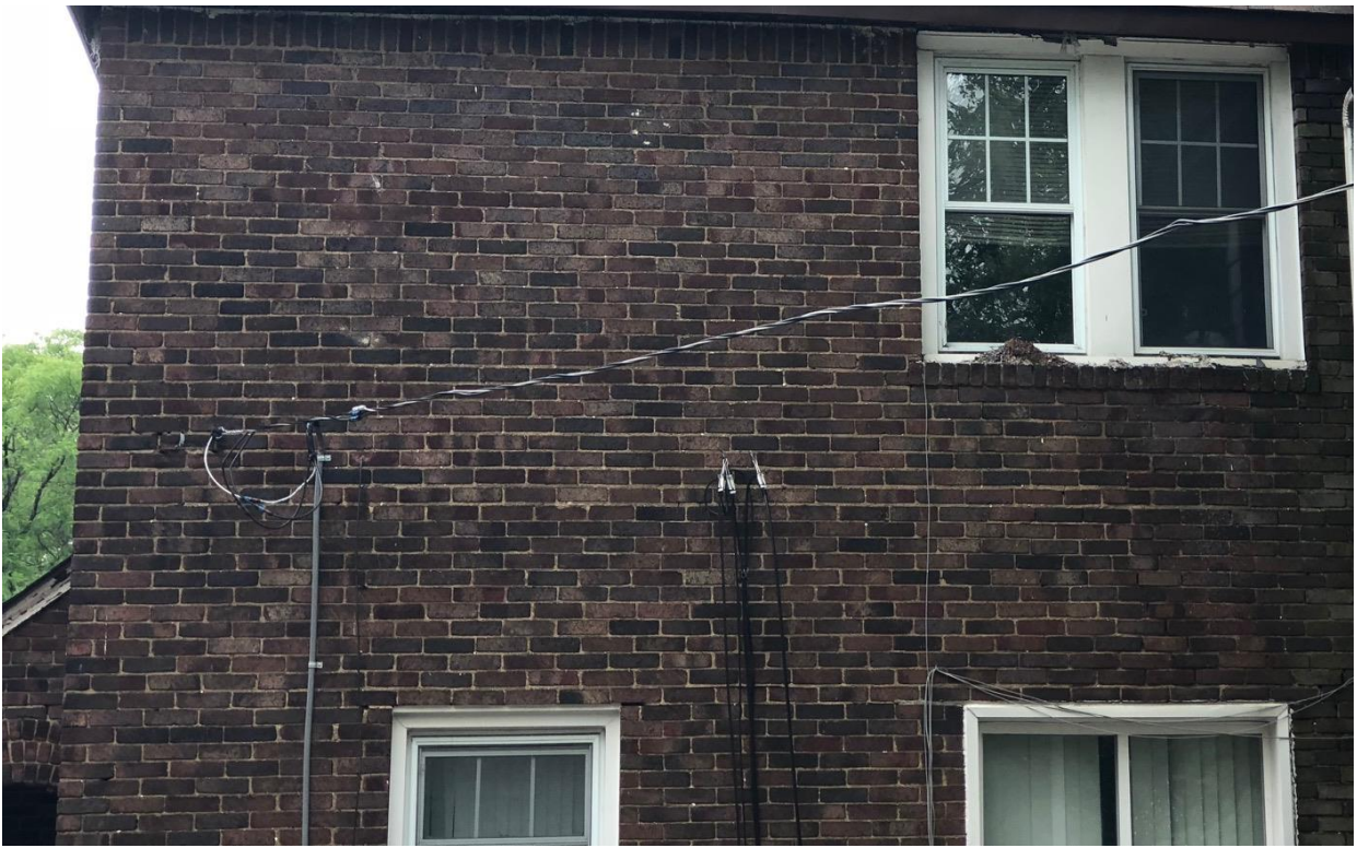
Rear wall, after the 2018 fire. Note that these windows are noncompatible, non-historic vinyl units which were approved for installation in 1985. Photo from applicant
