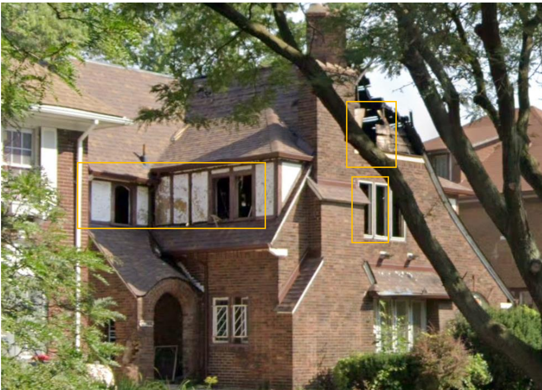
August 2018, after the fire. Window sash outlined in orange appear completely destroyed while their associated trim/casing/ remains. The rest of the windows also remain. Source, Google Streetview
