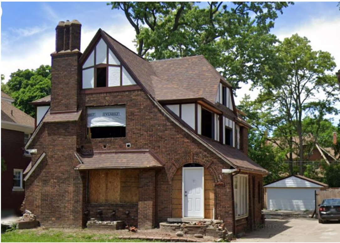
After the fire, 2019. Note that the second and attic story have been rebuilt, most windows and associated casing/brickmould have been removed to the rough opening, and front door sidelites have been removed. Garage siding has also been replaced per the 2018 COA. Source, Google Streetview
