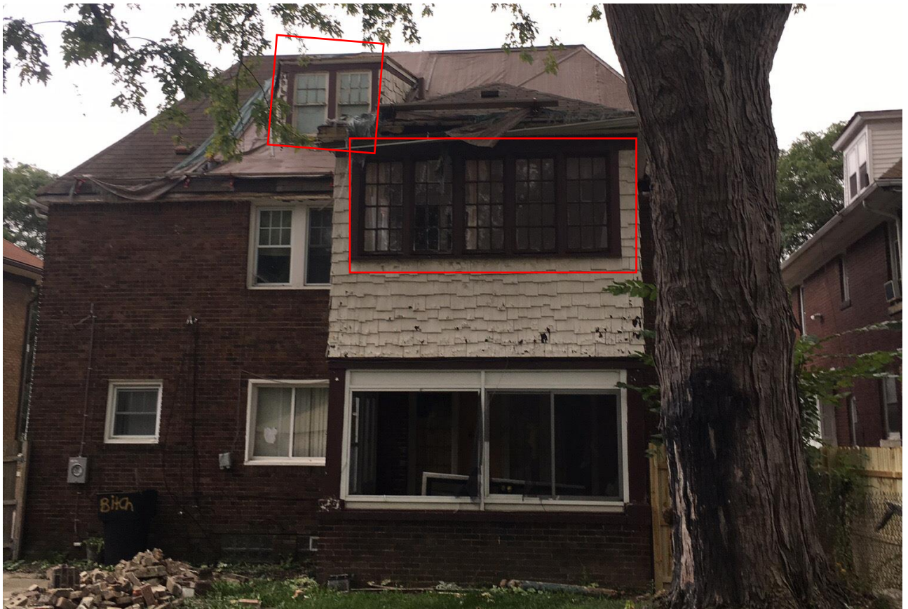
Photo taken in early 2018, prior to the fire. Wood sash casement windows outlined in red. Remaining windows are vinyl. Source, HDC files
