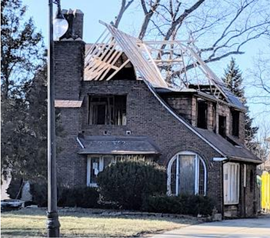
Late 2018, after the fire. Note that the rebuilding of the attic story is underway and all windows and associated casing/trim have been removed at the second story without HDC approval. Source, HDC files
