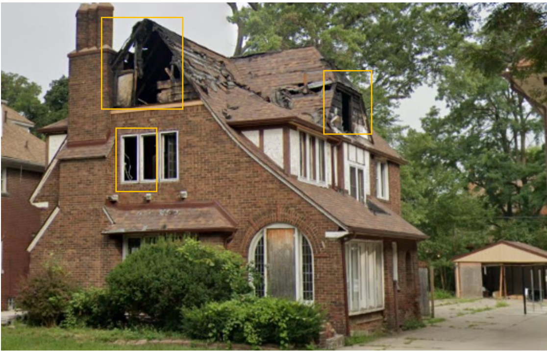
August 2018, after the fire. Note that most of the fire damage appears at the attic story and second story, west side. Windows sash and trim/casing at attic story outlined in orange appear completely destroyed. Two of the three casement window sash at the front façade, second story (outlined in orange) appear to be completely destroyed although the casing/trim remained. The rest appear to remain. The garage also appears not to have been fire damaged. Source. Google Streetview
