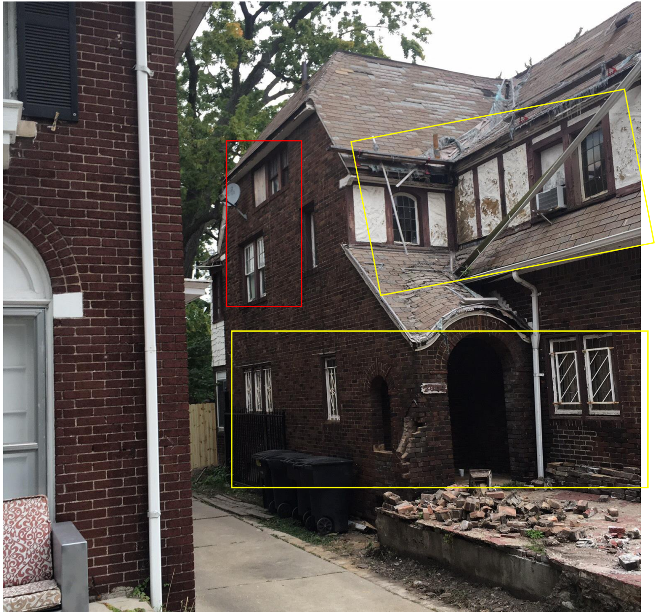
Photo taken in early 2018, prior to the fire. Note that all windows outlined in yellow are wood casement windows with leaded glass and those outlined in red are wood, double hung units. Source, HDC files.
