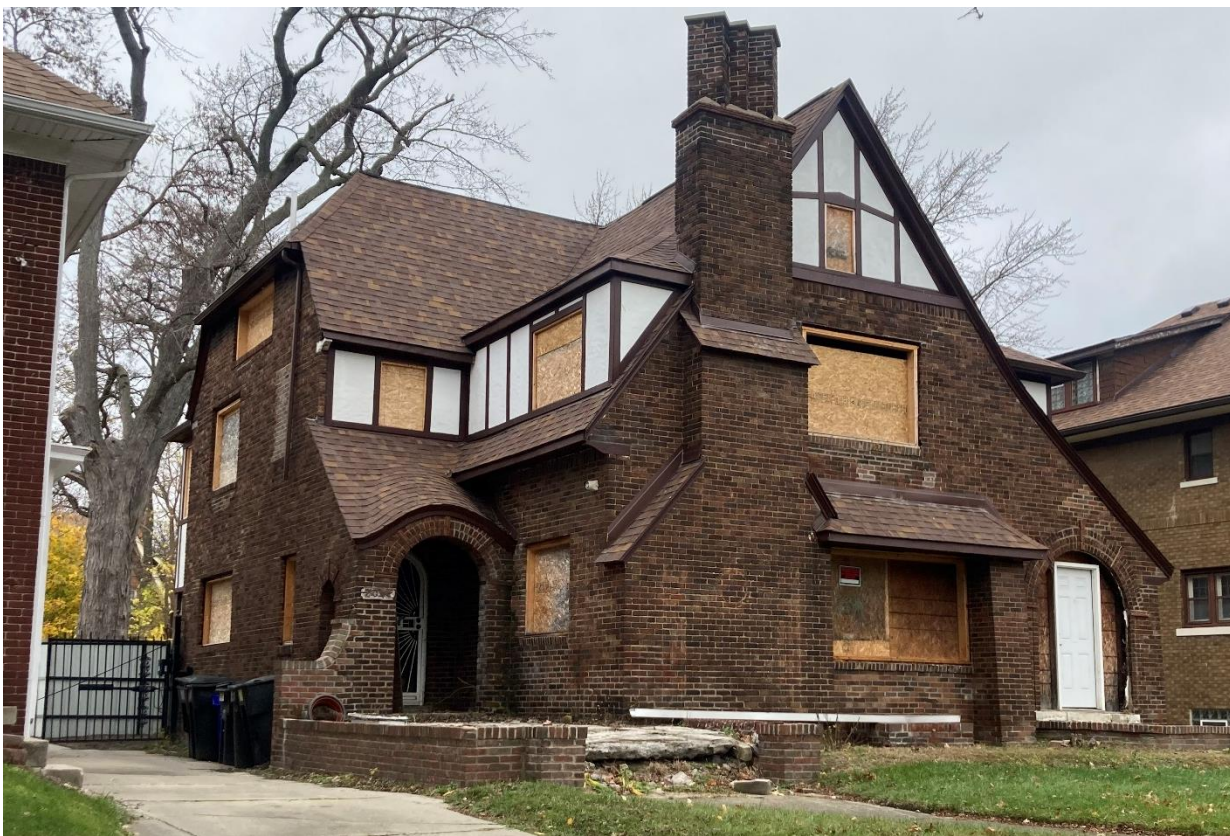
Current conditions. Note that the second and attic story have been rebuilt, most windows and associated casing/brickmould have been removed to the rough opening, and front door sidelites have been removed. Staff photo taken 4/25/2025
