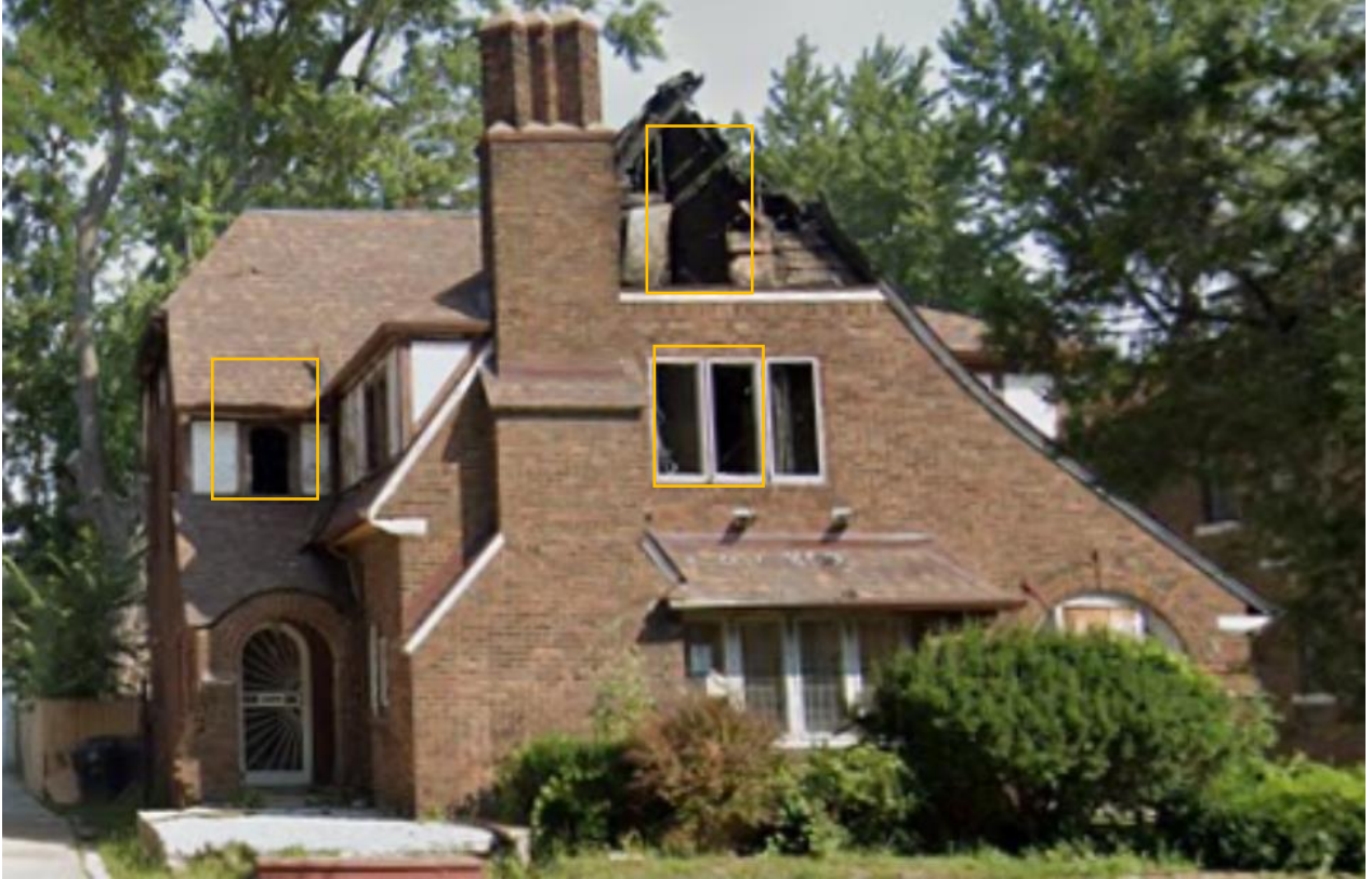
August 2018, after the fire. Window sash outlined in orange appear completely destroyed. The rest appear to remain. Source, Google Streetview
