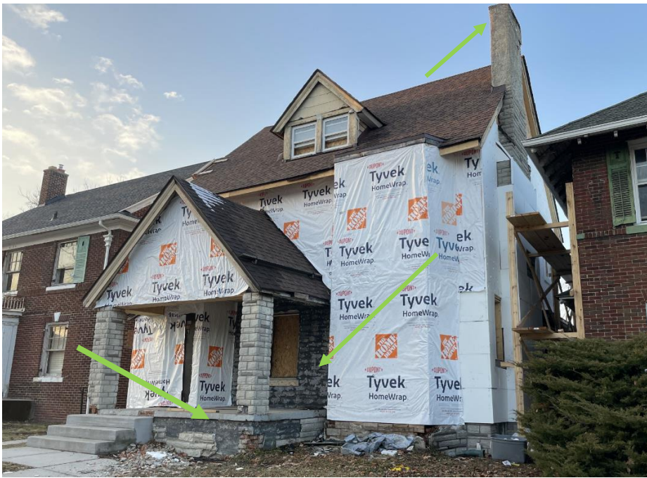
Conditions on 1/24/2023. Photo by HDC staff. Note stucco at chimney, porch floor and front wall (green arrows)
