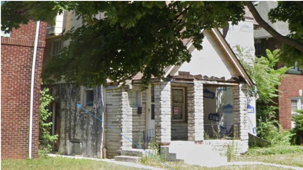
Conditions in 2020, per Google Streetview. Note where PermaStone has been removed to reveal original stucco finish at first story
