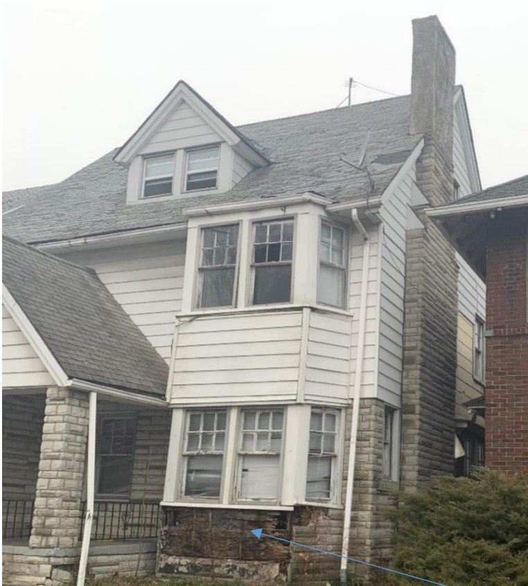
Photo taken in 2020 by owner. Note area where aluminum siding has fallen off, revealing synthetic shingle siding underneath.
