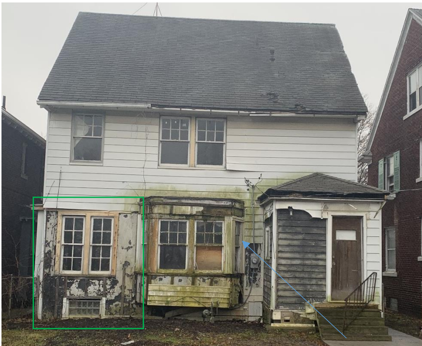
Rear, photo taken in 2020 by owner. Note apparent fire damage at first story. The area outlined in green shows original stucco finish at first story. Also, note that the fire has exposed the historic lapped wood siding at the siding at the hipped roof wing
