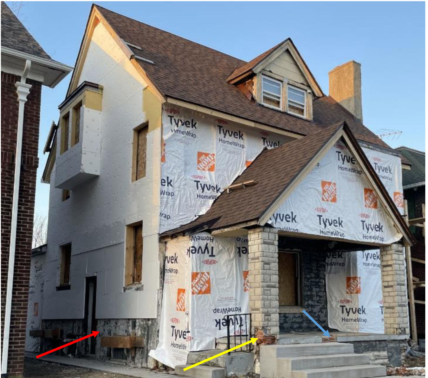
Conditions on 1/24/2023. Photo by HDC staff. Note that stucco remains beneath the current EIFS at the first story (red arrow). Also, note that the original masonry porch columns were masonry with stucco, as seen beneath the Permastone (yellow arrow). A centrally-located porch column had been removed by this point (blue arrow)
