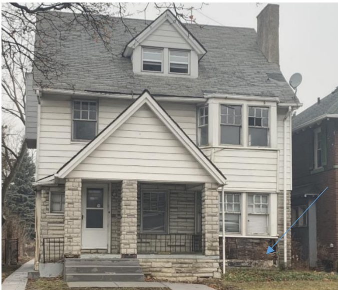
Front façade, 2020 photo taken by owner. Note area where Permastone has fallen off (indicated by blue arrow)
