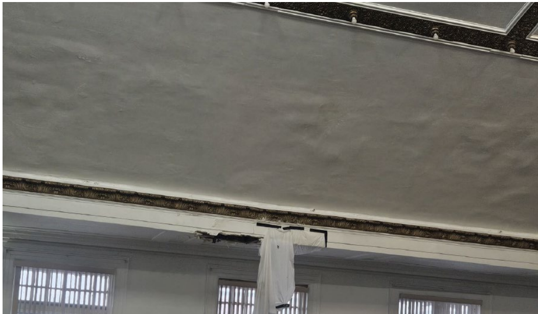
Photo from application showing interior water damage to plaster.
