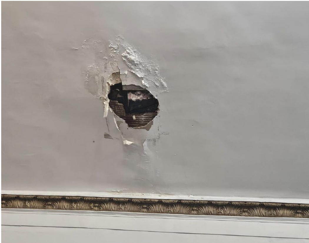
Photo from application showing interior water damage to plaster.
