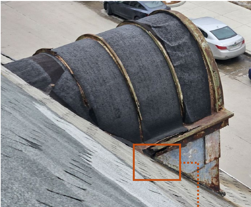
Photo from application showing deteriorated metal.
