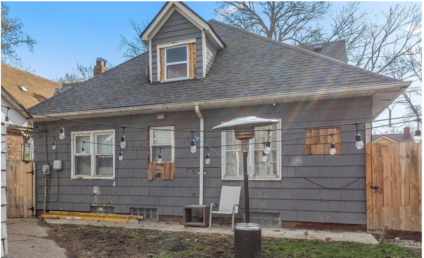
Rear wall showing unapproved vinyl window installation and window enclosure. Note that the one set of original 4/4, paired/mulled wood windows remained at this time (indicated by blue arrow). The windows have since been removed. Photo taken in 6/2024 by former applicant.
