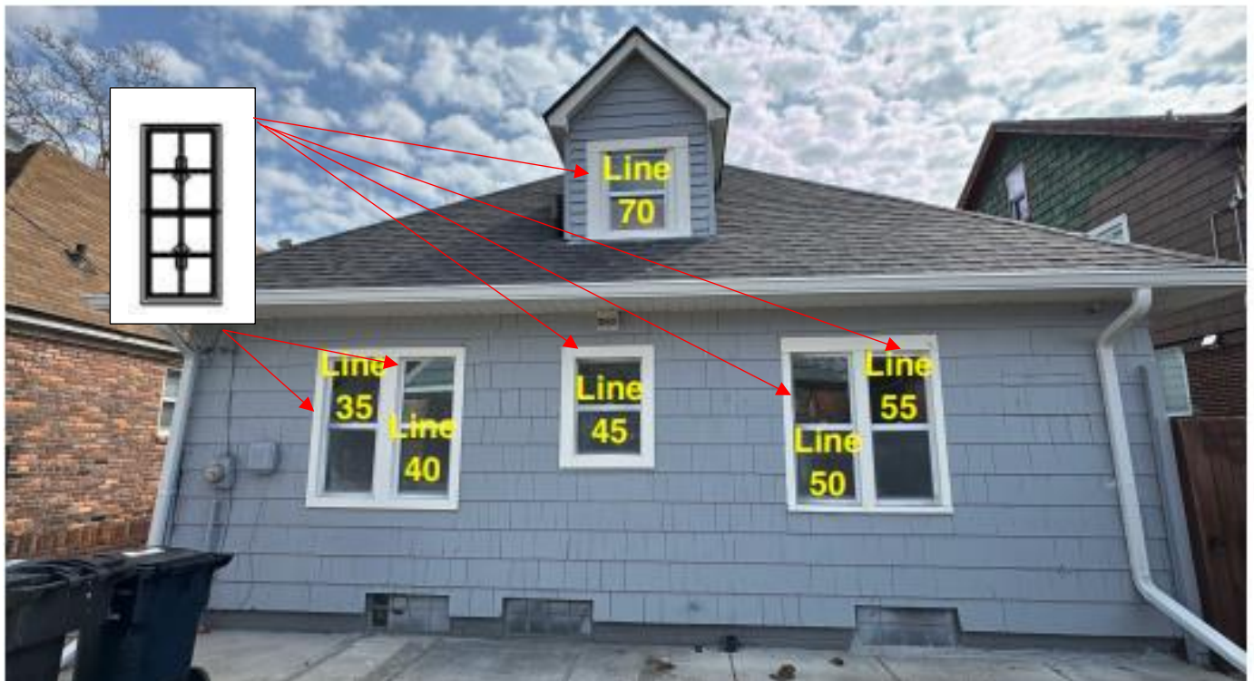
Rear elevation. Six (6), 4/4, double-hung, aluminum clad wood sash windows to be installed. Existing wood trim will be retained. Note that vinyl siding appears to have been installed at the dormer; the opening for window labeled “Line 45” has been partially infilled and covered with singles; and an opening to the right of the window labeled “Line 55” has been infilled and covered with shingles.
