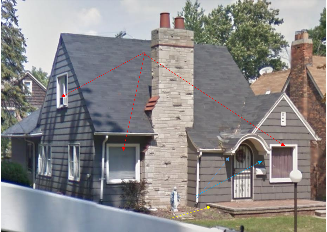
Appearance in 2013. Source, Google Streetview. Between 1999 and 2013 new vinyl windows (indicated by red arrows) and porch (indicated by yellow arrow) were installed. Also, the historic brackets at the front door canopy were removed (indicated by blue arrow).
