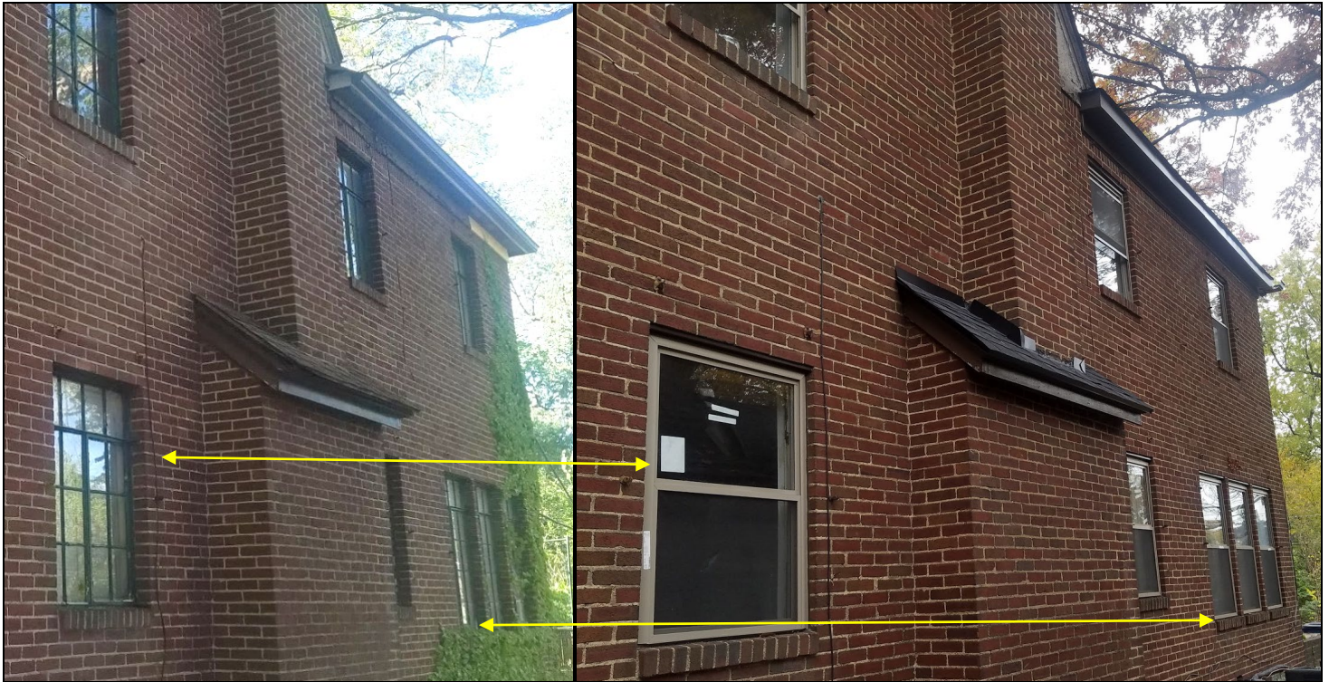
The depth of the “before” steel windows is quite evident and clearly offers a relief from the masonry wall. The replacement windows are minimally set back in the window opening, and from a distance, appear to be in plane and a part of the exterior wall. Applicant photos.
