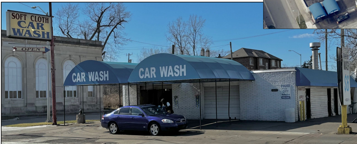
Looking northwest, the photo shows the front of the building facing E. Jefferson.
