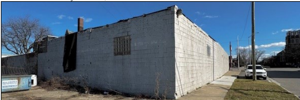
North (rear) and west walls; concrete block and glass block.
