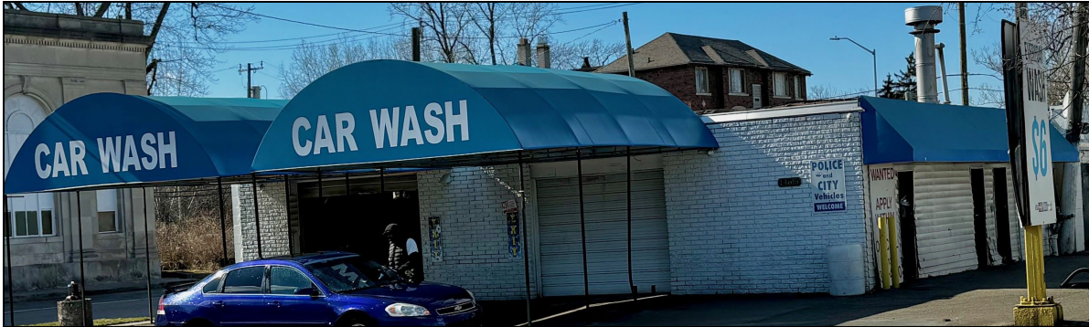
Façade facing East Jefferson; brick veneer. Staff photos, March 2025.
