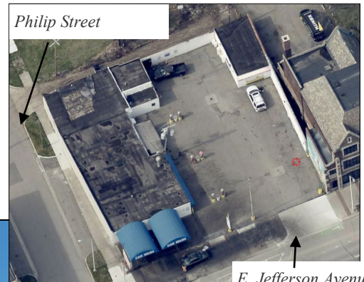
E. Jefferson Avenue Aerial View, EagleView 2024.
