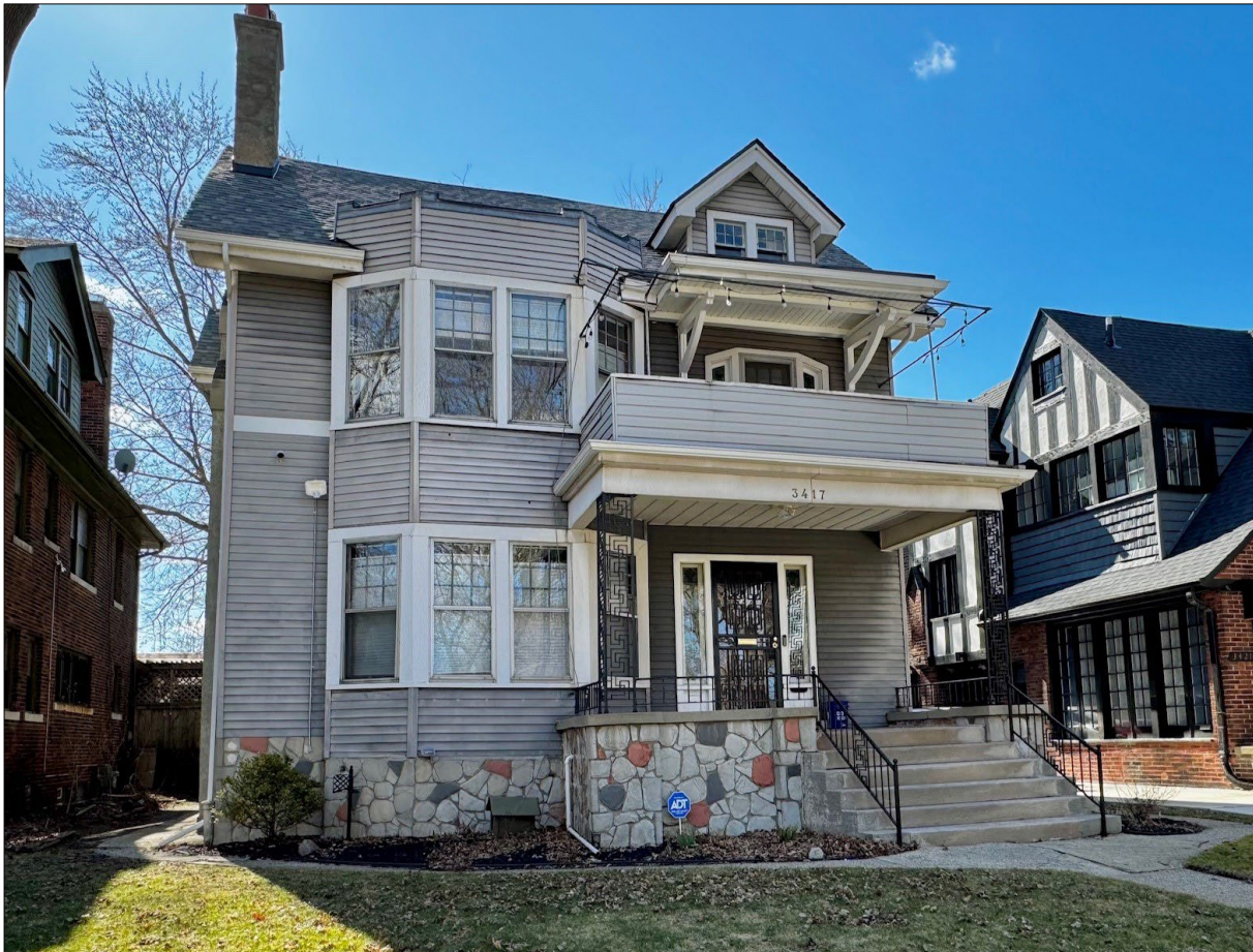
Facade, east-facing wall. Staff photo, March 26, 2025.
