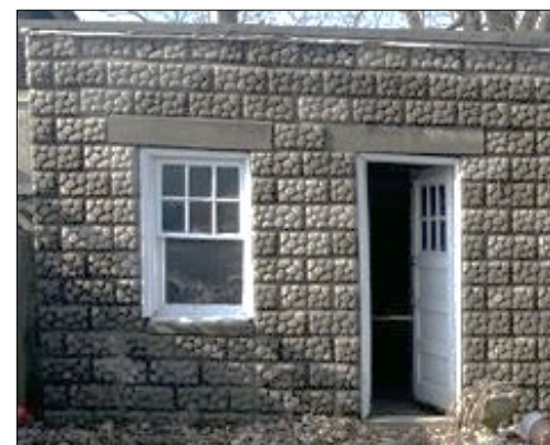
Exterior view of wall at left.
