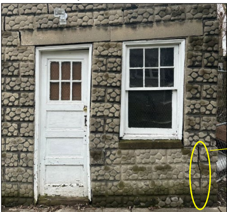
Exterior view of wall at right.
