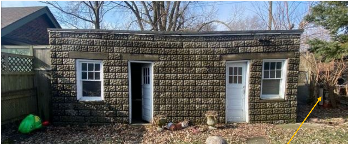
East wall of garage facing the rear yard and back of house. The third bay is essentially missing, with only one wall fully intact. Applicant photo.
