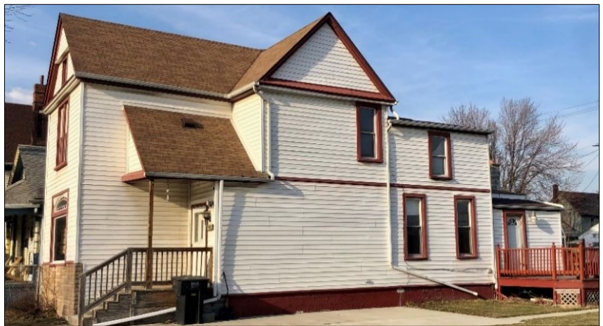
Left and above: Existing conditions at the time of the Commission's first review of the property (24-00031, March 13, 2024 mtg.). Vinyl siding covered the walls and the windows were trimmed in aluminum coil. Staff photos, February 21, 2024.
