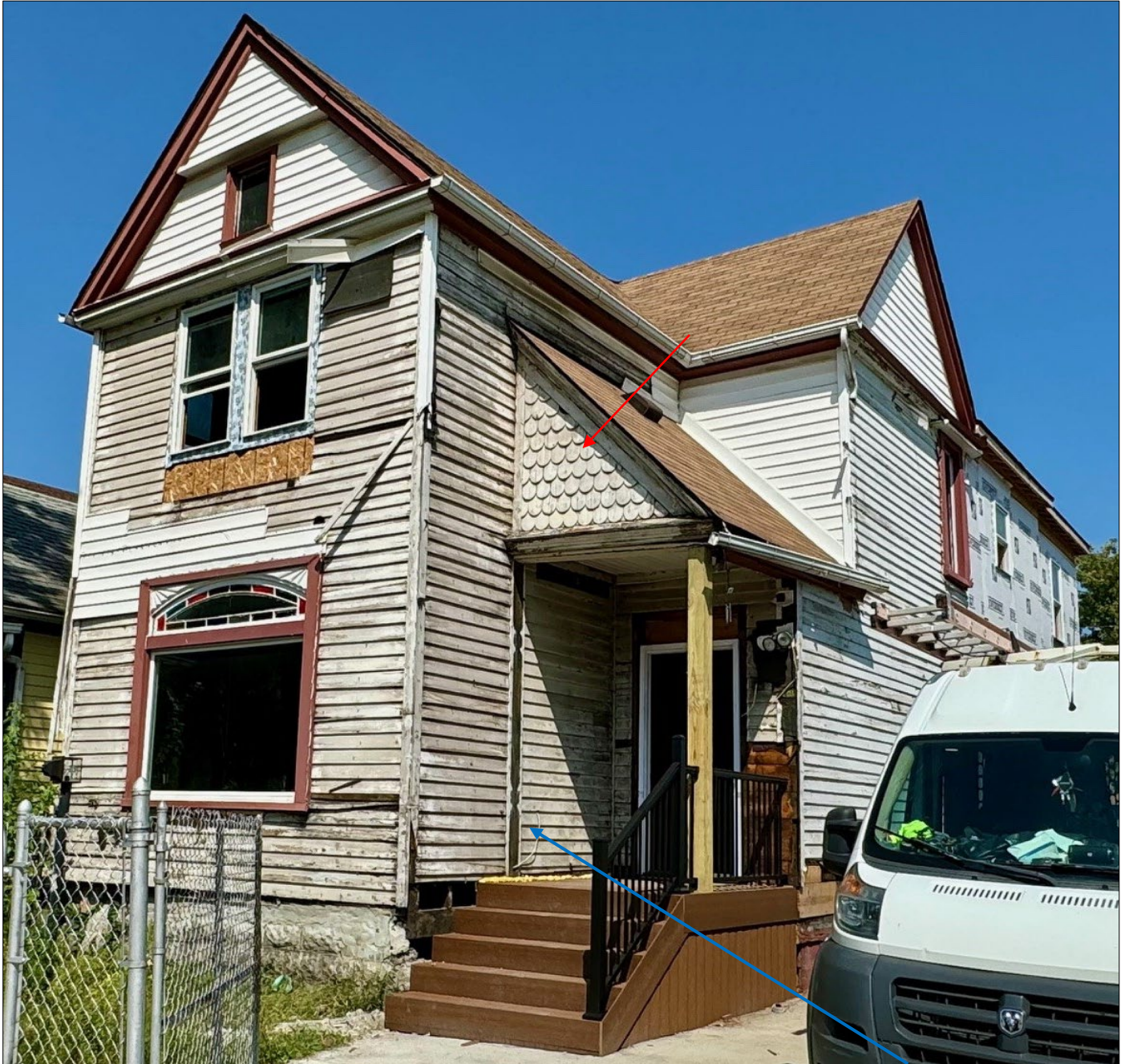
Front and side walls. Notice the scallop siding that was uncovered at the porch (red arrow), as well as the ghost image/profile of the original porch post against the house's wall (blue arrow). Staff photo, August 2024.
