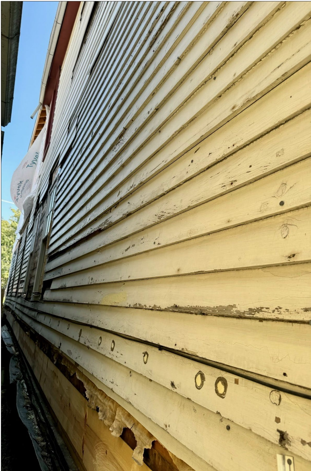
Detail - north side wall. The contractor invited staff to closely inspect the lap siding; it was intact and in very good condition. Staff photo, August 2024.
