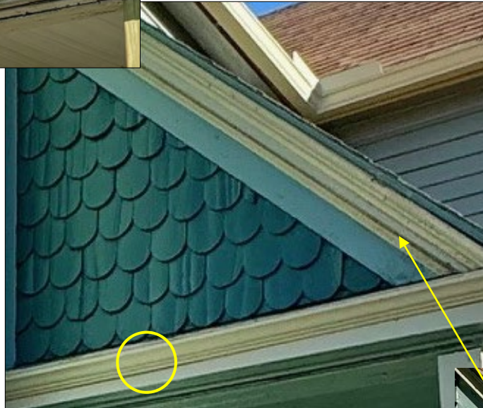
January 6, 2025. The reflective sheen of the paint shows the smooth surface of the historic scallop panels (where cracks aren't present). Note the highly profiled bargeboard at the angled roof remains, similar to the historic condition (at left), but it appears as though the lower wide bargeboard has been replaced with a narrower product. Staff photo.
