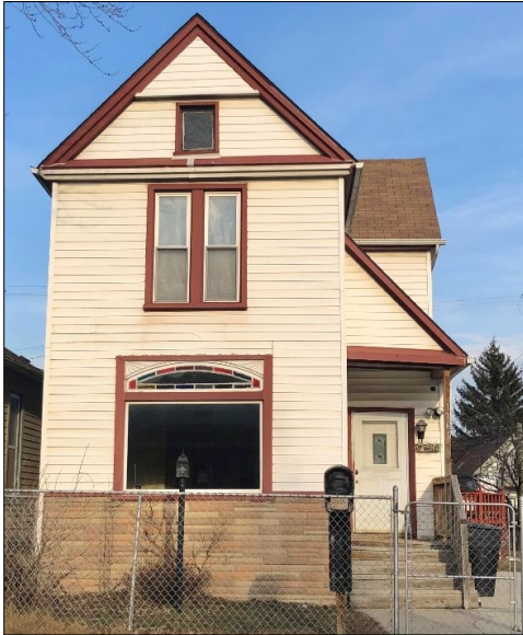
Left and above: Existing conditions at the time of the Commission's first review of the property (24-00031, March 13, 2024 mtg.). Vinyl siding covered the walls and the windows were trimmed in aluminum coil. Staff photos, February 21, 2024.
