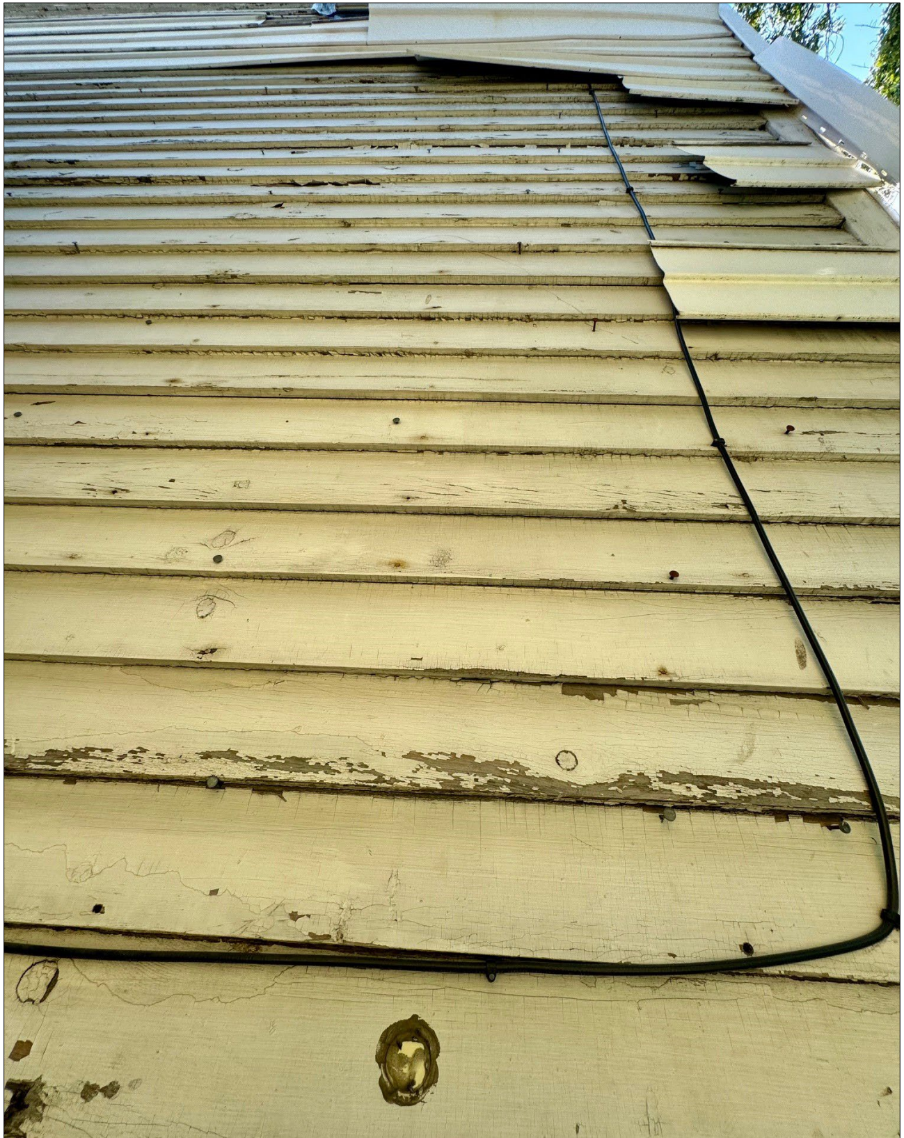
Another partial view of the north wall, near the front of the house. The historic siding had only a small number of nail holes that would need to be filled. Staff photo, August 2024.
