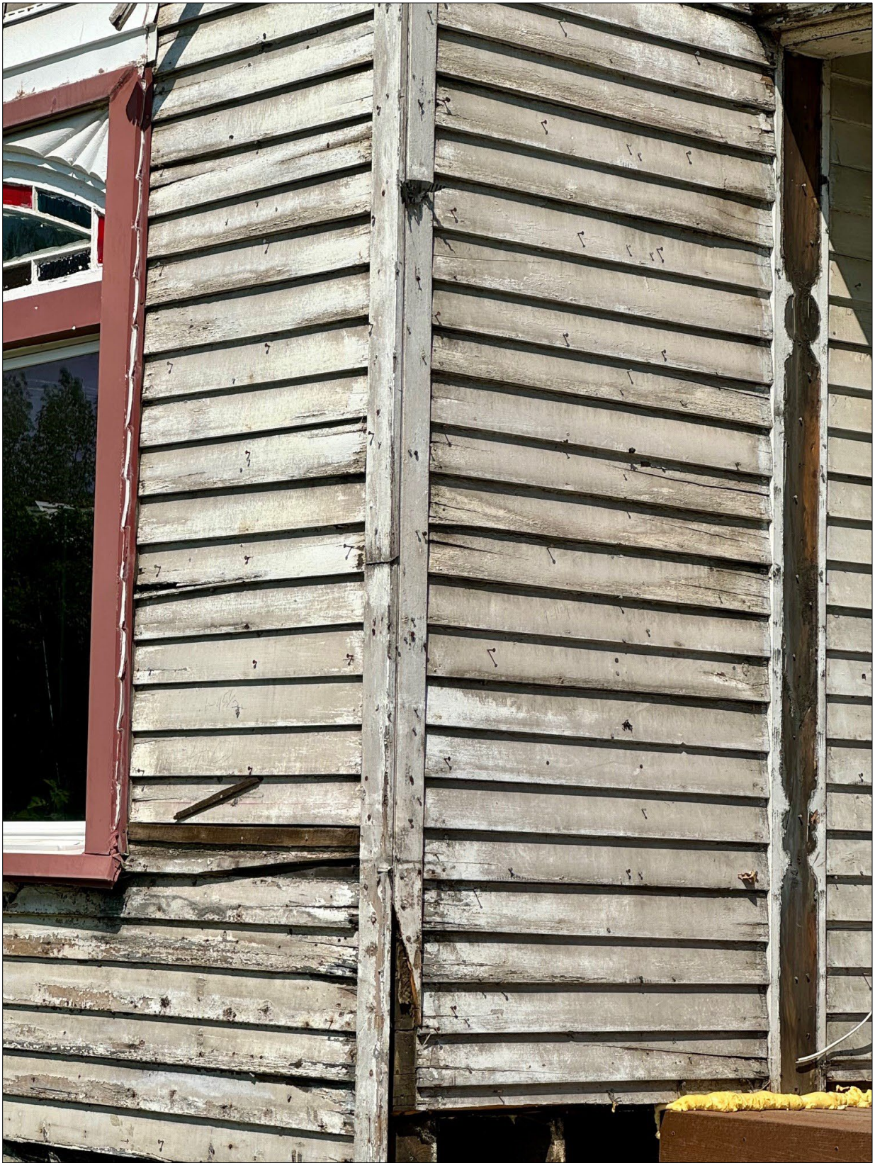
This detail image of the southwest front corner of the house near the porch shows mostly intact lap siding with minimal deterioration (repairable deterioration is most evident where the lap siding met the corner boards). The aluminum coil stock remains on the windows casings at the front window. Staff photo. August 2024.
