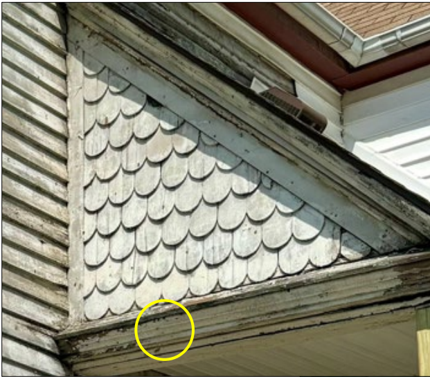
August 2024. This photo shows that the historic scallop siding had a similar smooth surface texture as the adjacent historic lap siding. The scallop siding is uniformly framed with flat trim, and then two outer sections had thickly dimensioned bargeboard trim applied to meet the roof/porch ceiling. Staff photo.
