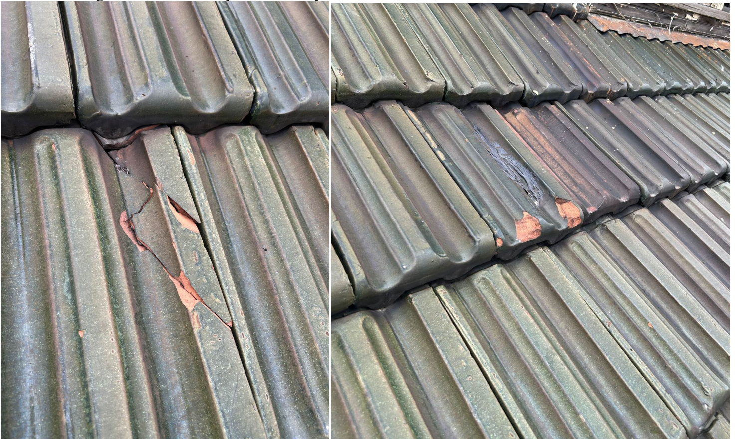
Applicant photos of cracked tiles.
