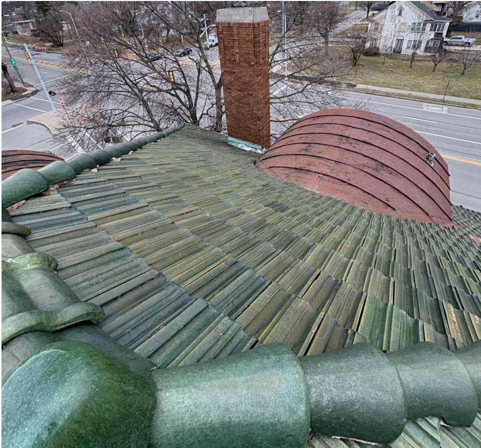
Applicant photo. View of east-facing roof, looking toward the Chicago and Hamilton intersection. The ridge and hip trim pieces appear to be in great shape.
