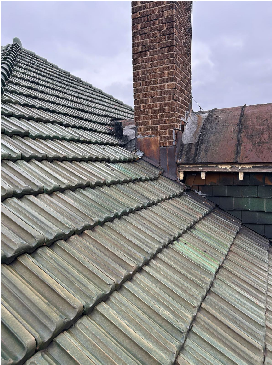
Applicant photo, flat green tiles at dormer wall are visible. The flashing at the chimney appears to need replacement.
