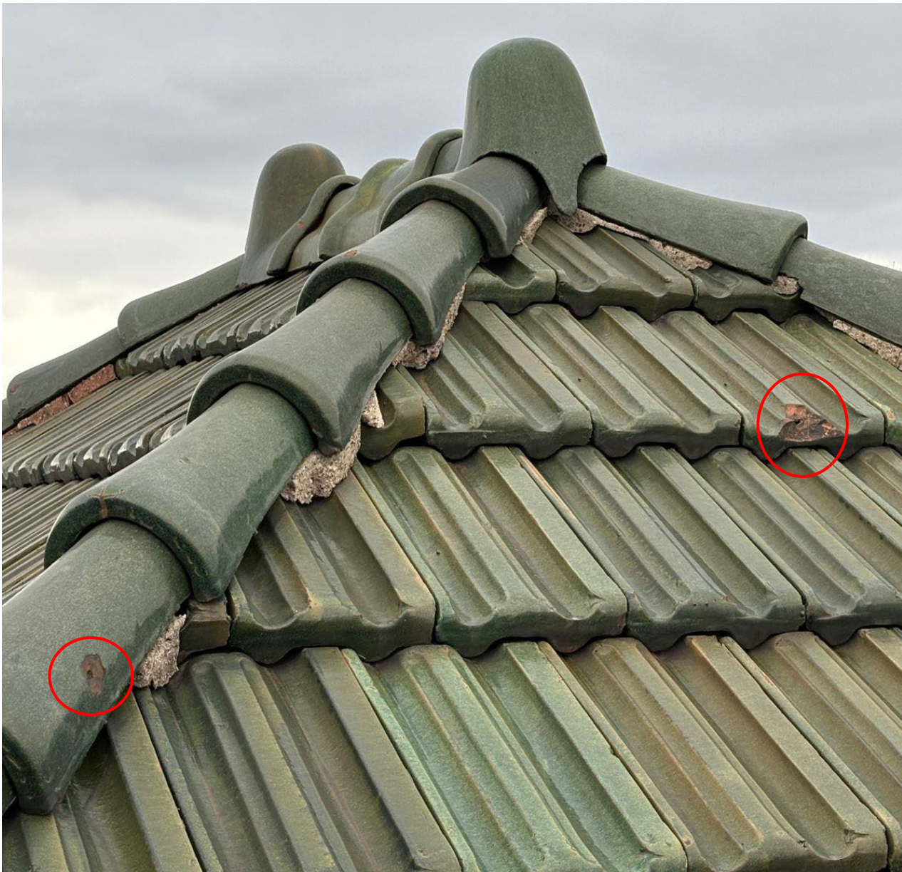
This is a view of the highly dimensional top of the roof. Within this expanse of tile, it appears there is one tile with a broken edge, and one ridge cap with a chipped finish.
