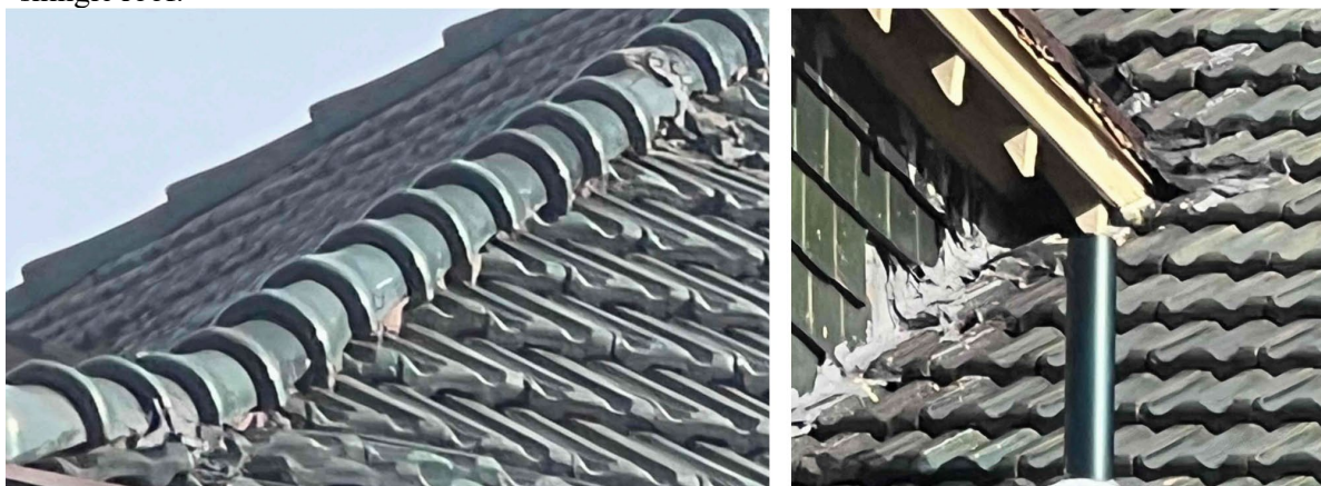
Photos, from application documents, showing loose tiles and patched areas. Flat green tiles clad the dormer walls.
