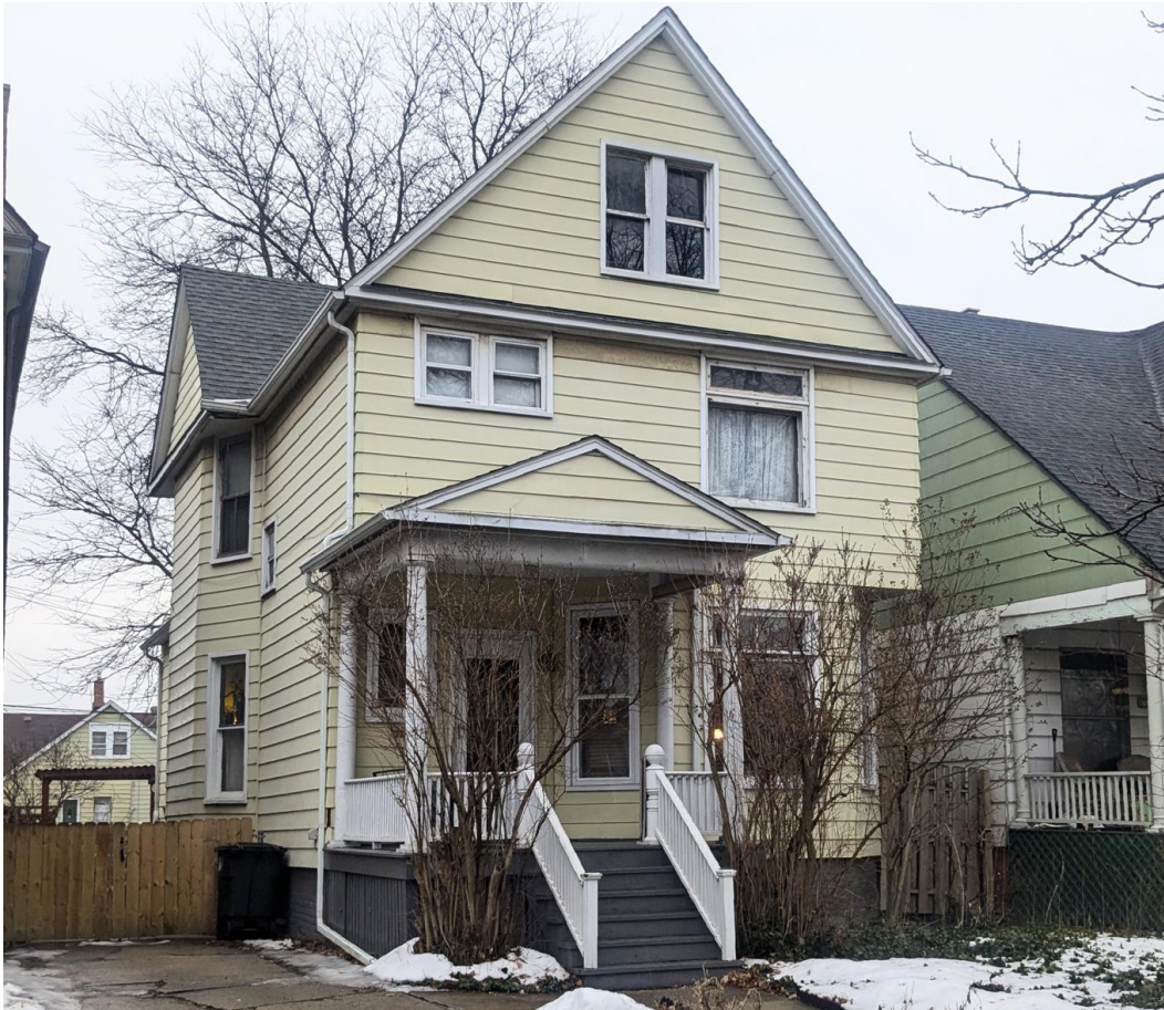
1817 Leverette viewed from the north. February 2025 photo by staff.
