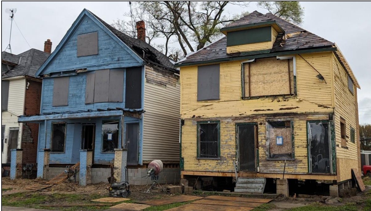
Existing conditions, April 2024. HDC staff photo.
