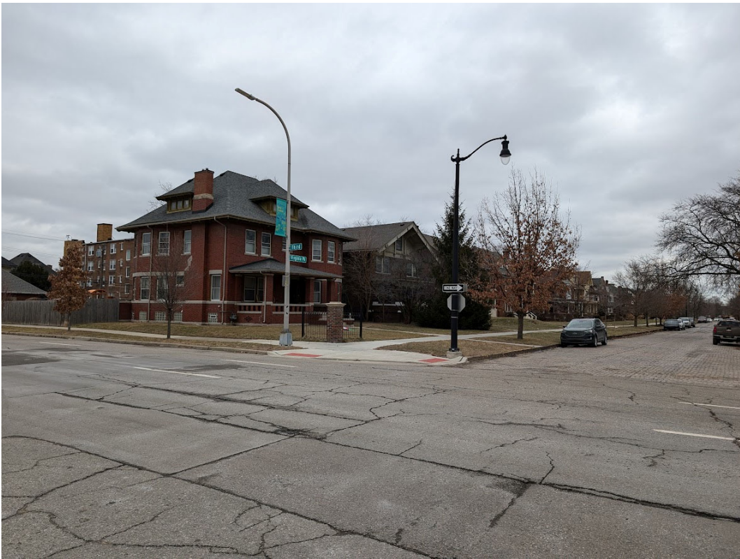
View to the east showing historical context of Virginia Park Avenue, north side, east of Third. Staff photo, February 4, 2025.
