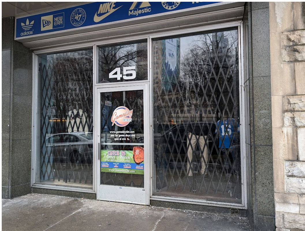
View of 23-31 East Adams, showing typical post-war storefront at Adams elevation. Staff photo, January 31, 2025.
