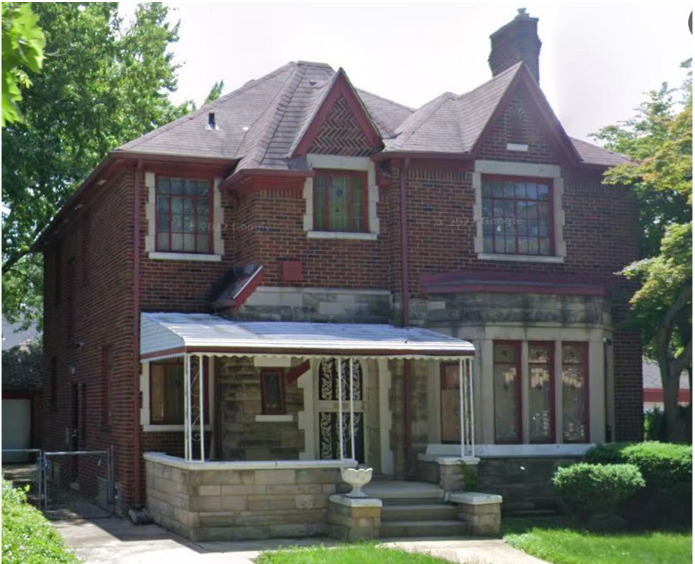
2022 Google Street View photo showing historic windows.
