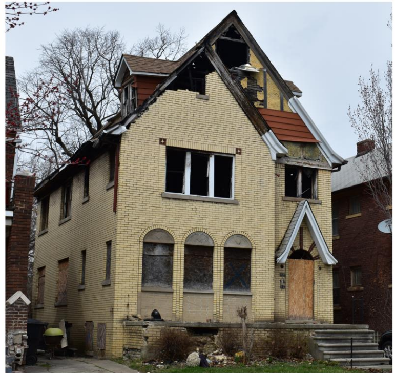
Fire damage and exposed stucco and half timbering seen in 2009 Google Maps photo (left) and 2019 staff photo (right).
