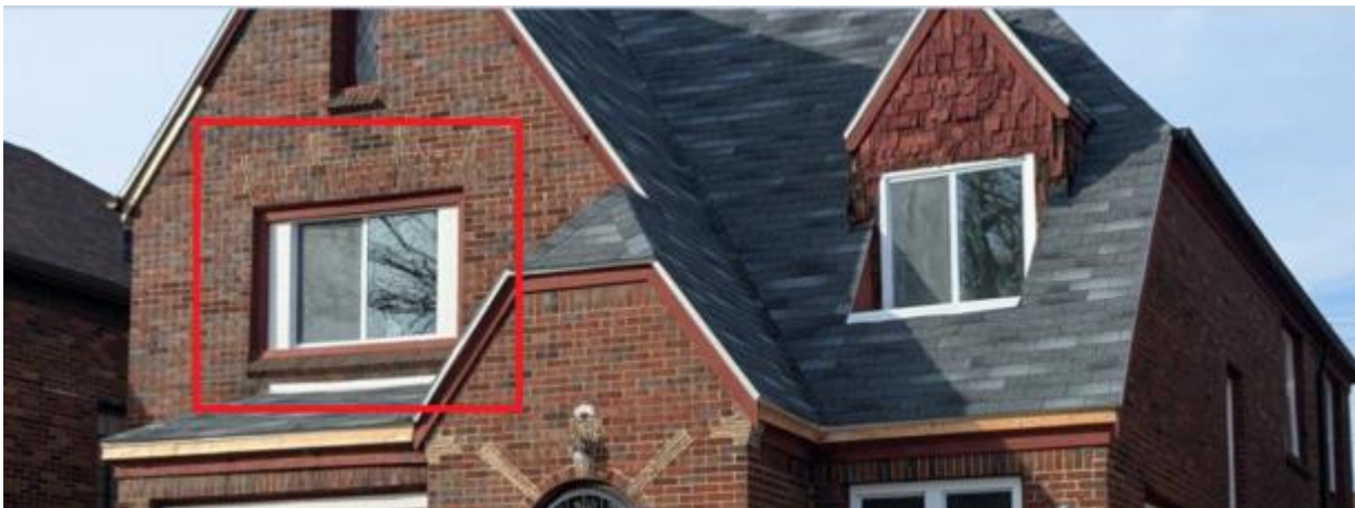
Red box indicates the windows that would appropriately be replaced with the three-unit, mullioned windows as depicted above.
