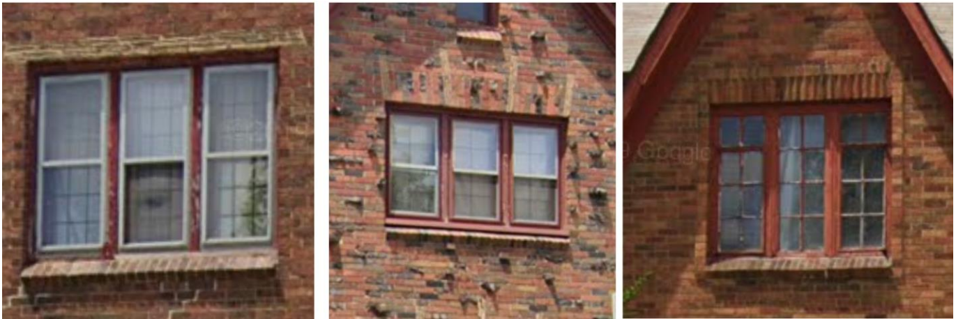
Google Maps images showing examples of mullioned, second-story, wall-gable windows on the same block as the subject property. Such window groupings are very common and are an important part of the district’s character.
