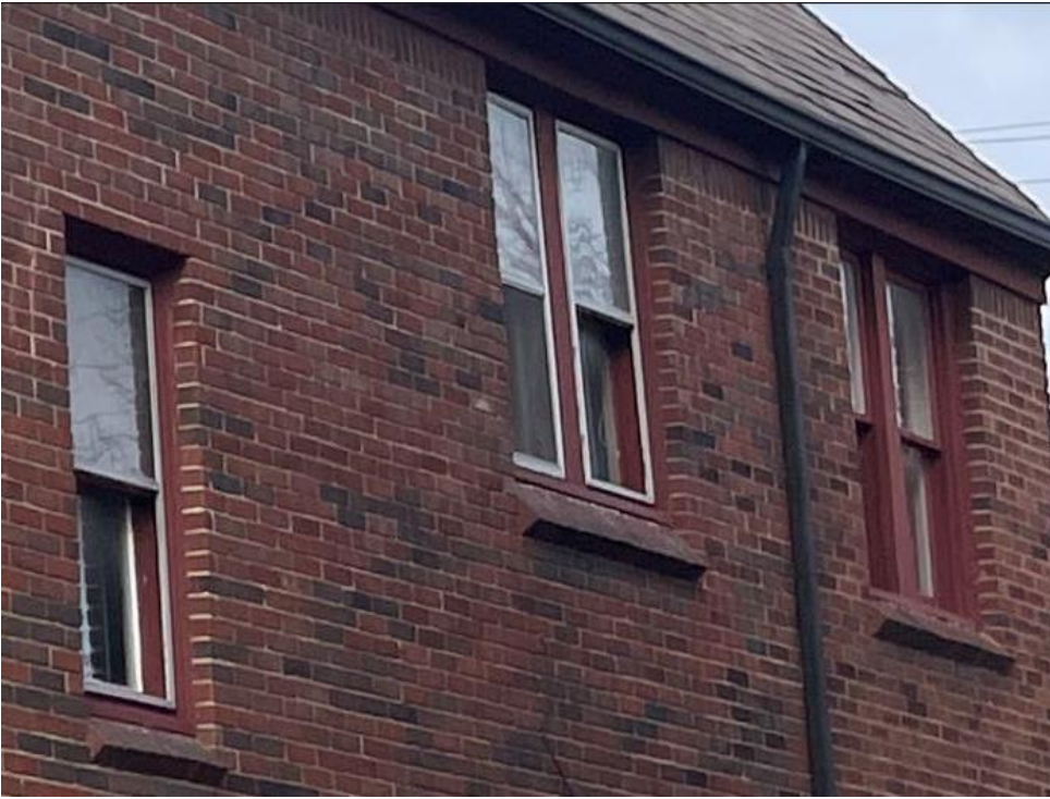
West elevation, second floor. February 2024 photo by staff.
