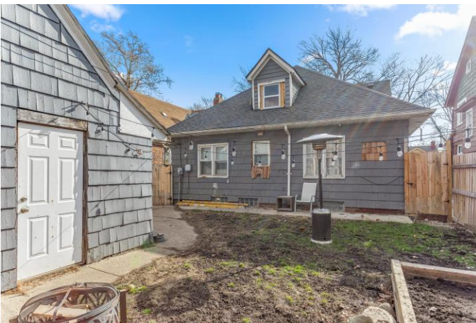
Image from 2024 application documents showing the two remaining historic windows on the house (partly hidden behind the patio heater).
