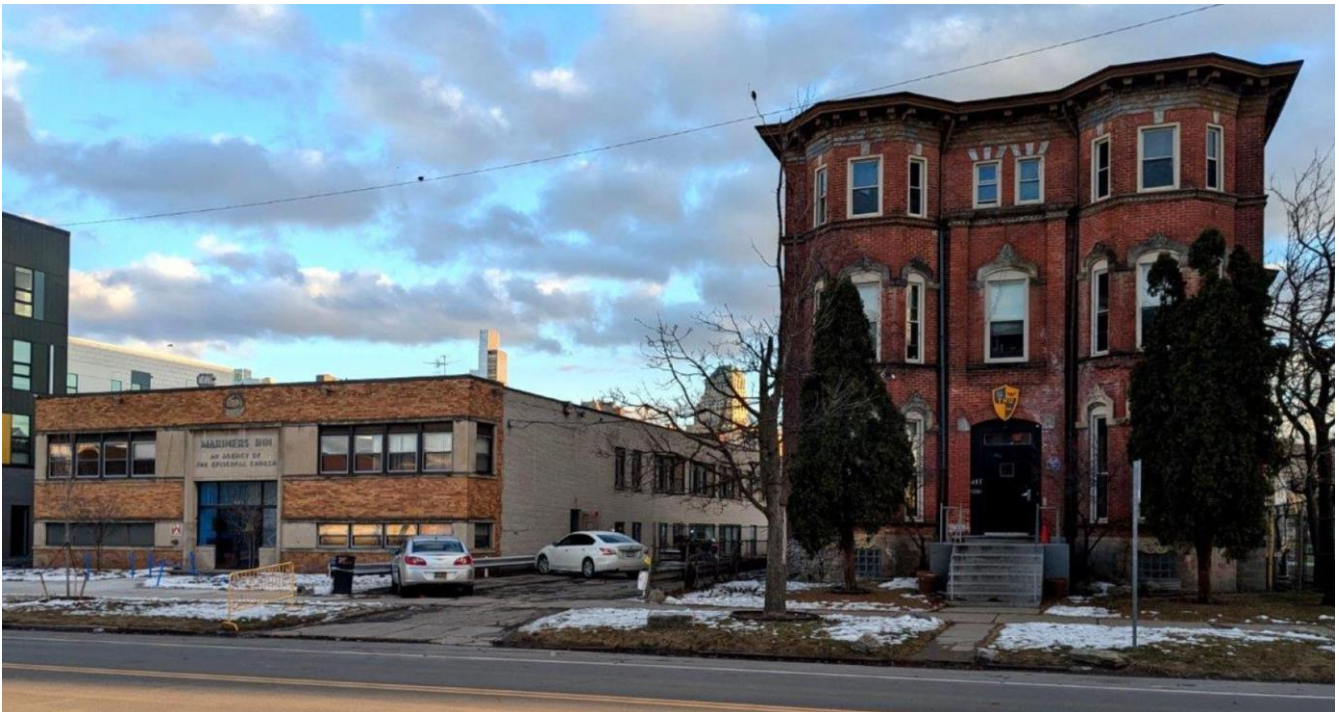
The subject properties, viewed from the north. January 2025 photo by staff.
