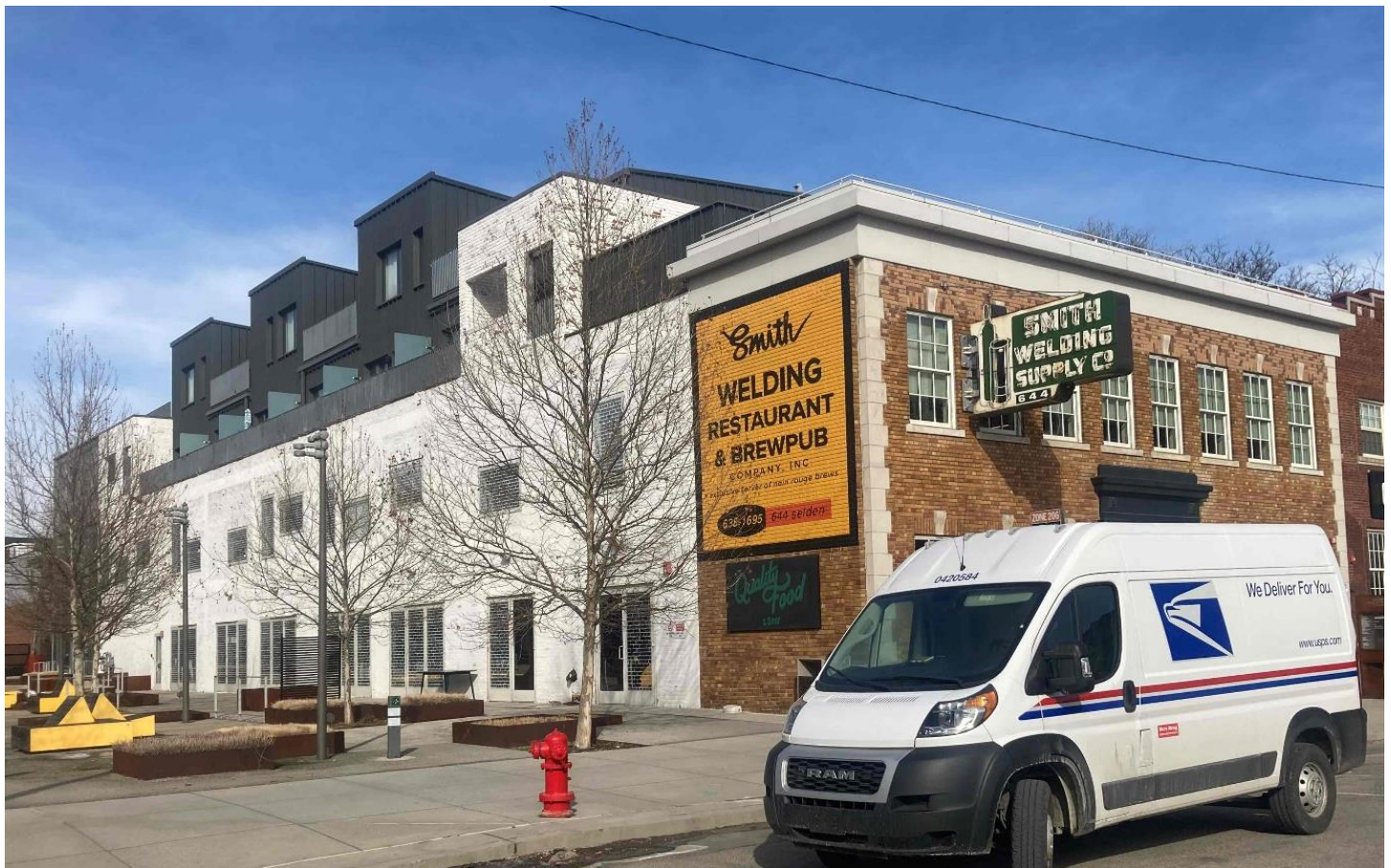
644 Selden, current appearance. Photo by staff.
