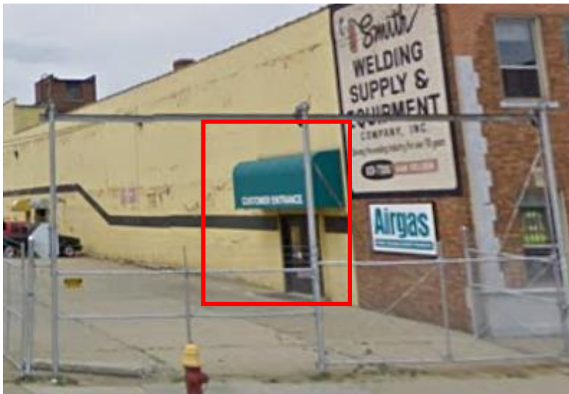
Location of proposed new primary entry doors and tile cladding. Google Streetview image dating from 2007. This opening was widened to accommodate the current set of paired aluminum doors during the 2019 rehabilitation
