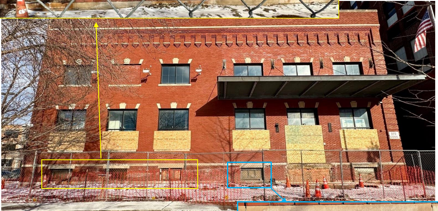
The five basement window openings are visible in the above photo. Two of the openings are covered with panels (metal or wood); the remaining three openings have historic window sash exposed. At right is a close view of one of the steel windows. Staff photos, January 24, 2025.
