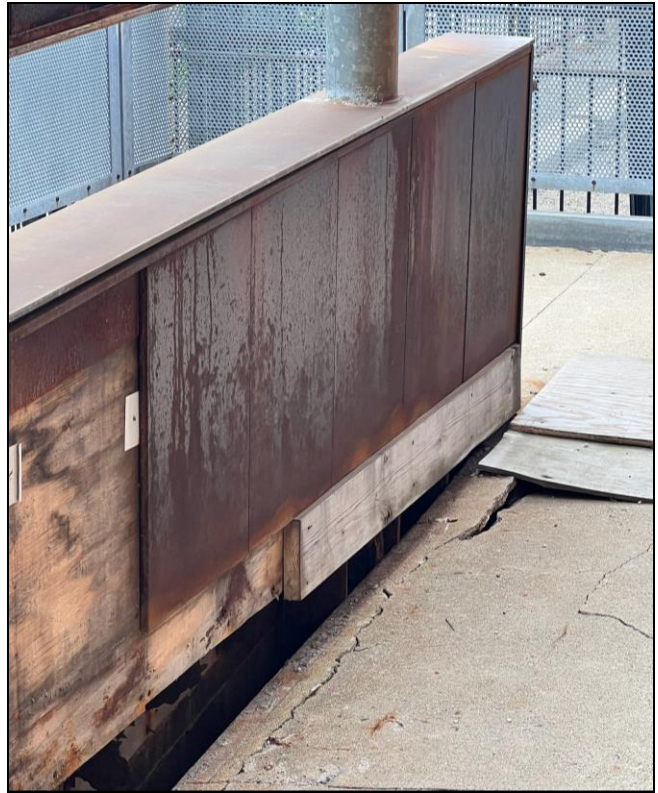
This view shows metal panels that were placed within the basement window openings.
