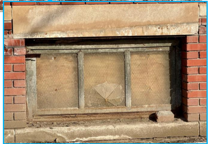
The five basement window openings are visible in the above photo. Two of the openings are covered with panels (metal or wood); the remaining three openings have historic window sash exposed. At right is a close view of one of the steel windows. Staff photos, January 24, 2025.
