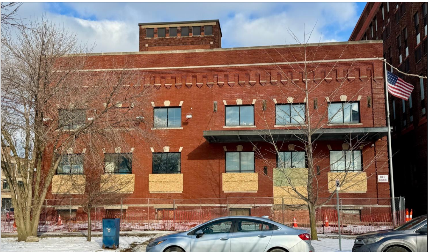
Facade facing Second Avenue. HDC staff photo, January 24, 2025.
