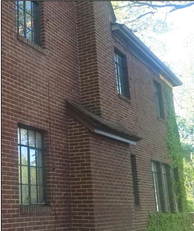
The depth of the "before" steel windows is quite evident and clearly offers a relief from the masonry wall. The replacement windows are minimally set back in the window opening, and from a distance, appear to be in plane and a part of the exterior wall.
