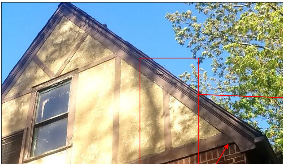
This undated applicant photo shows an intact highly profiled rake board on the west-facing gable wall. Note the curved edge at the bottom right of the photo. This detail common on English Revival houses may have been removed upon covering the rake board with aluminum.
