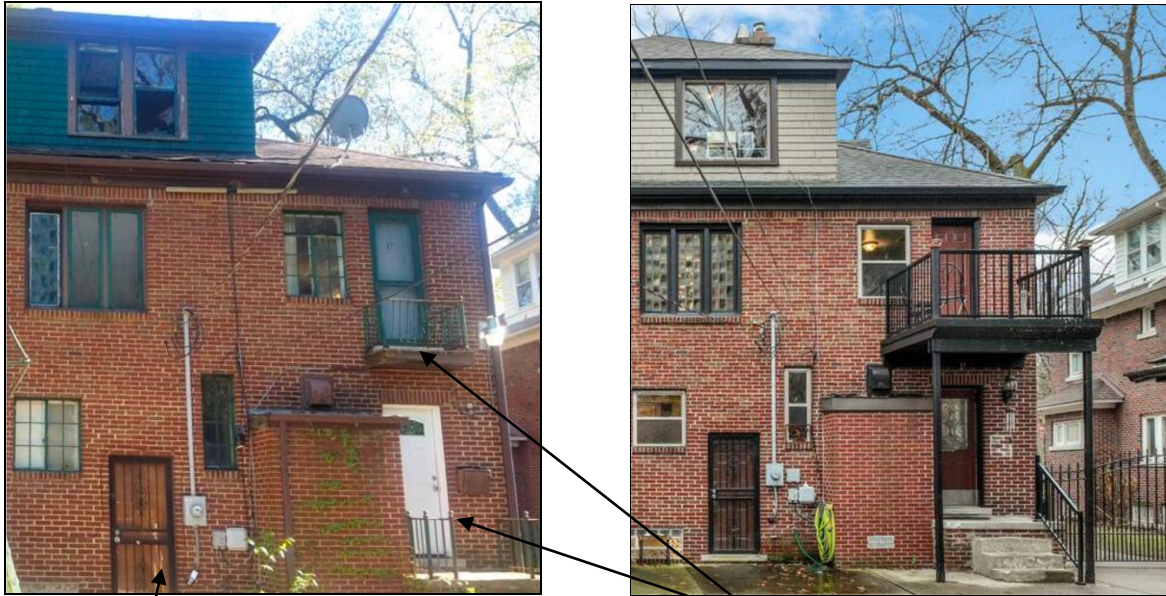
Above left: The wood door appears to be a solid, utilitarian door, and the two white non-historic doors are not appropriate for the architectural style of the house. The current replacement doors have minimal styling, and the brown color is compatible with the house's architectural design.
