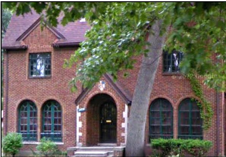
Above: Façade. Google street view, August 2015.
