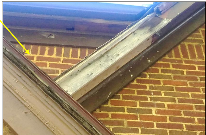
This applicant photo with the aluminum removed, shows an intact and highly profiled rake board at the front entry (at left), and a partial repair of the rake board within the large gable wall (middle). The soffit and wood trim (top) have small, but repairable holes.
