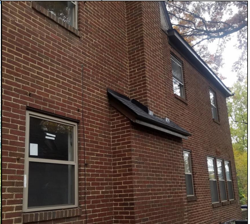
The depth of the "before" steel windows is quite evident and clearly offers a relief from the masonry wall. The replacement windows are minimally set back in the window opening, and from a distance, appear to be in plane and a part of the exterior wall.
