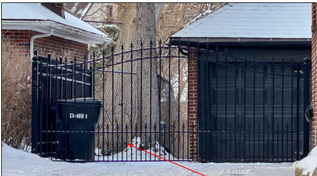
Staff photo from sidewalk, January 24, 2025. It appears that the black fencing was installed at the property line and a section of new chain link fencing was installed to bridge the space between the new black fence and an existing chain link fence.
