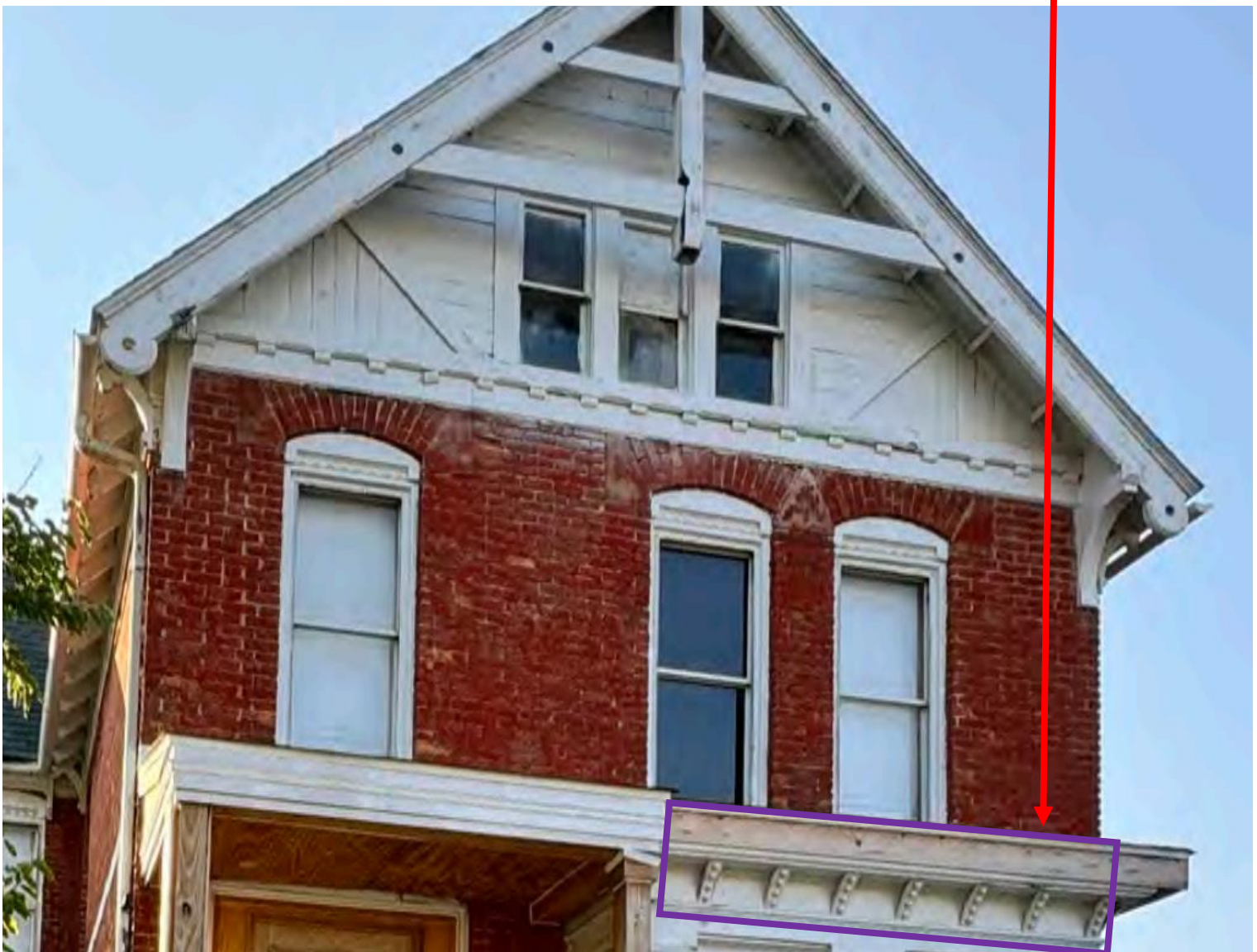
Front façade, current appearance. Note that the east side porch's decorative details match those at the front bay window. Specifically, the brackets at the porch soffit/eave area match those at the front facade bay (outlined in purple). Provided by applicant
