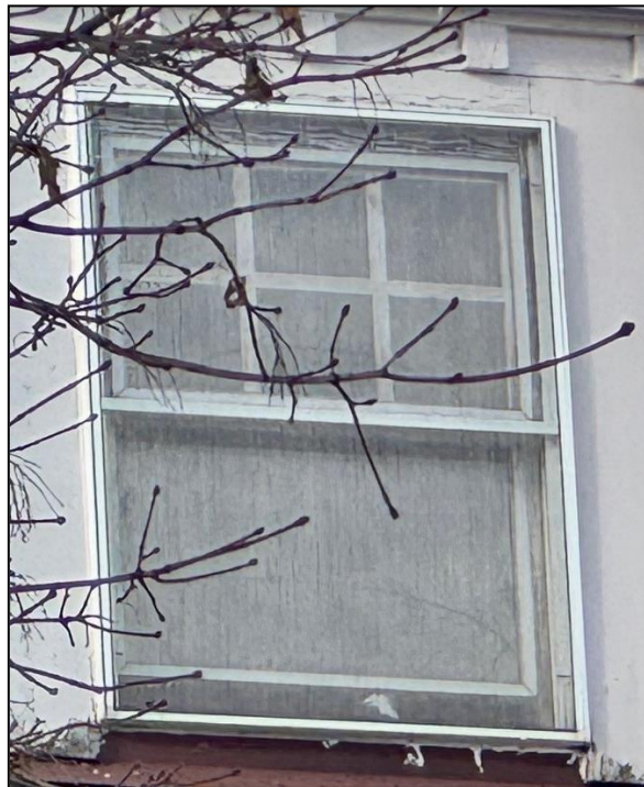
This photo is of a dormer on the rear of the house. The wood sash is recessed within the window opening. (This placement is slightly obscured by the protruding aluminum screen frame.) It also appears that replacement glass/flat grids have been installed within the wood sash frame. Staff photo, January 24, 2025.
