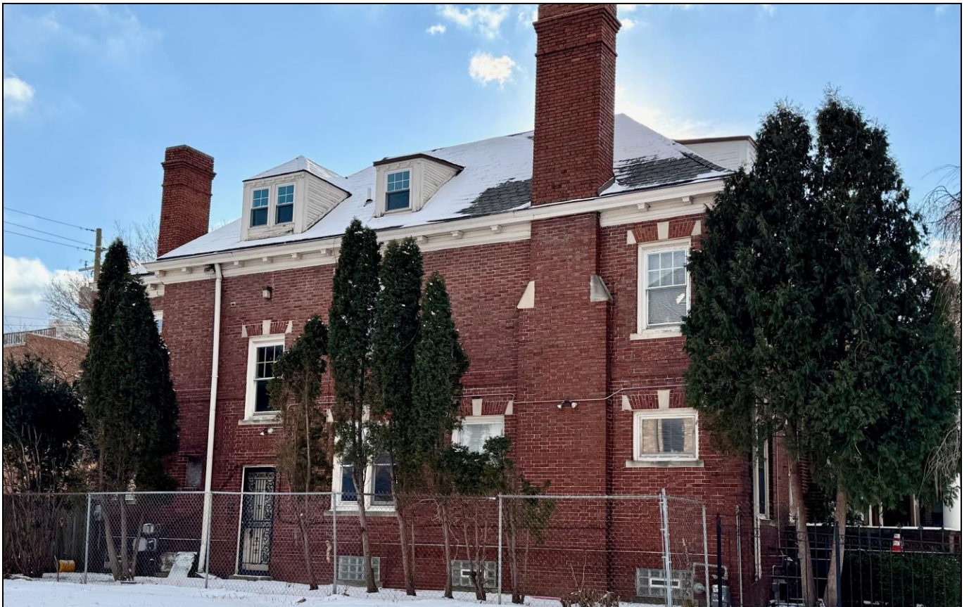
East – side wall. The three windows within the two dormers are vinyl replacement units. Staff photo.
