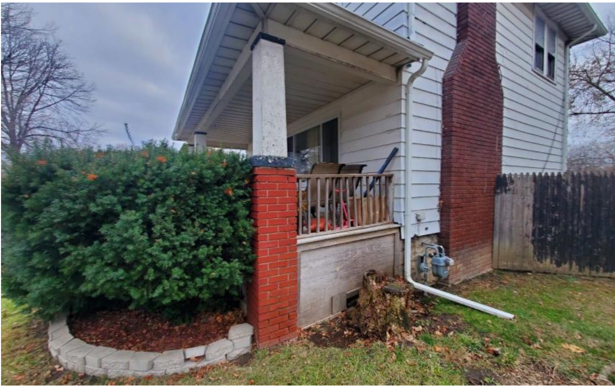
14258 Ashton. Photo by applicant, facing northeast, showing current condition of porch.
