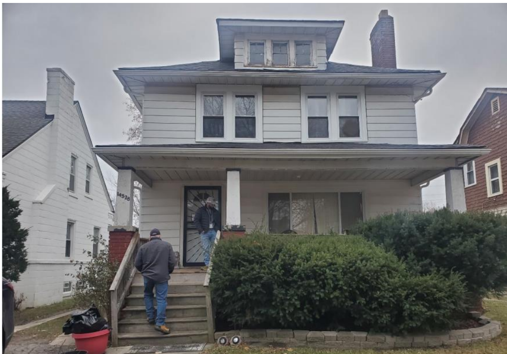
14528 Ashton, facing east. Photo by applicant showing current conditions. Note the wood railing, steps, skirting, and decking which were added without HDC approval in 2016. Also, note the non-historic masonry paver edging at foundation planting
