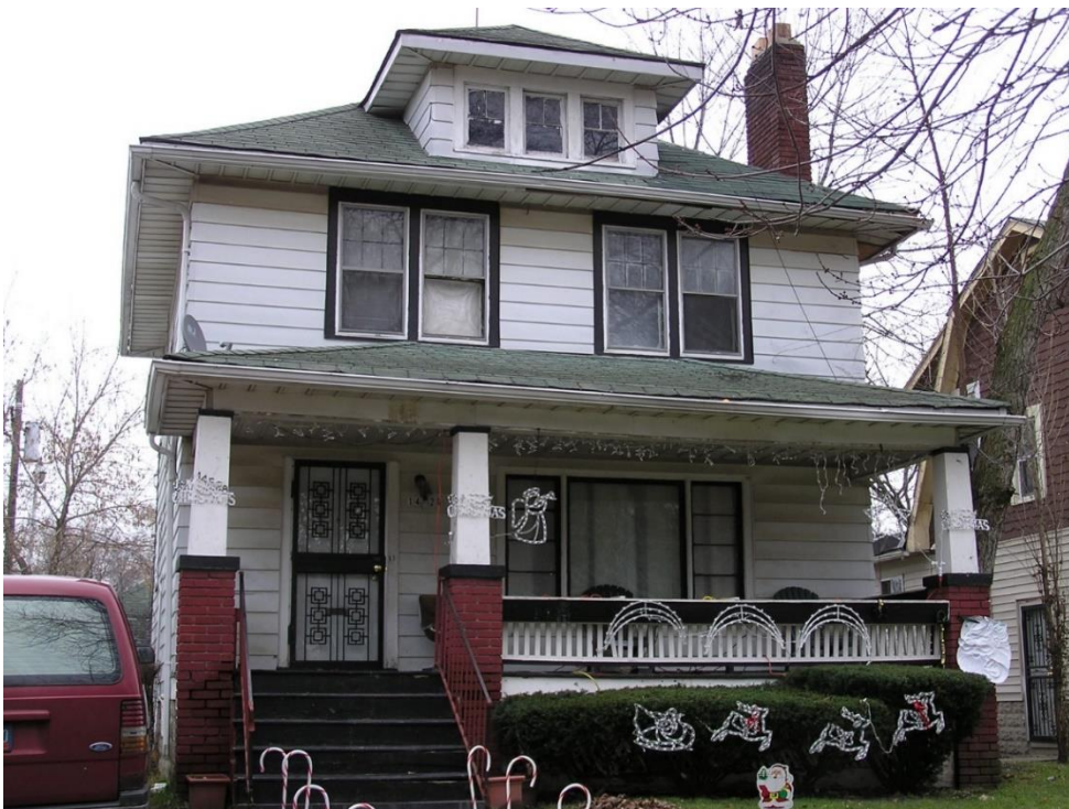
14528 Ashton, designation photo facing east. HDAB staff, 2008. Note wood railing decking, and steps. Handrails are metal.
