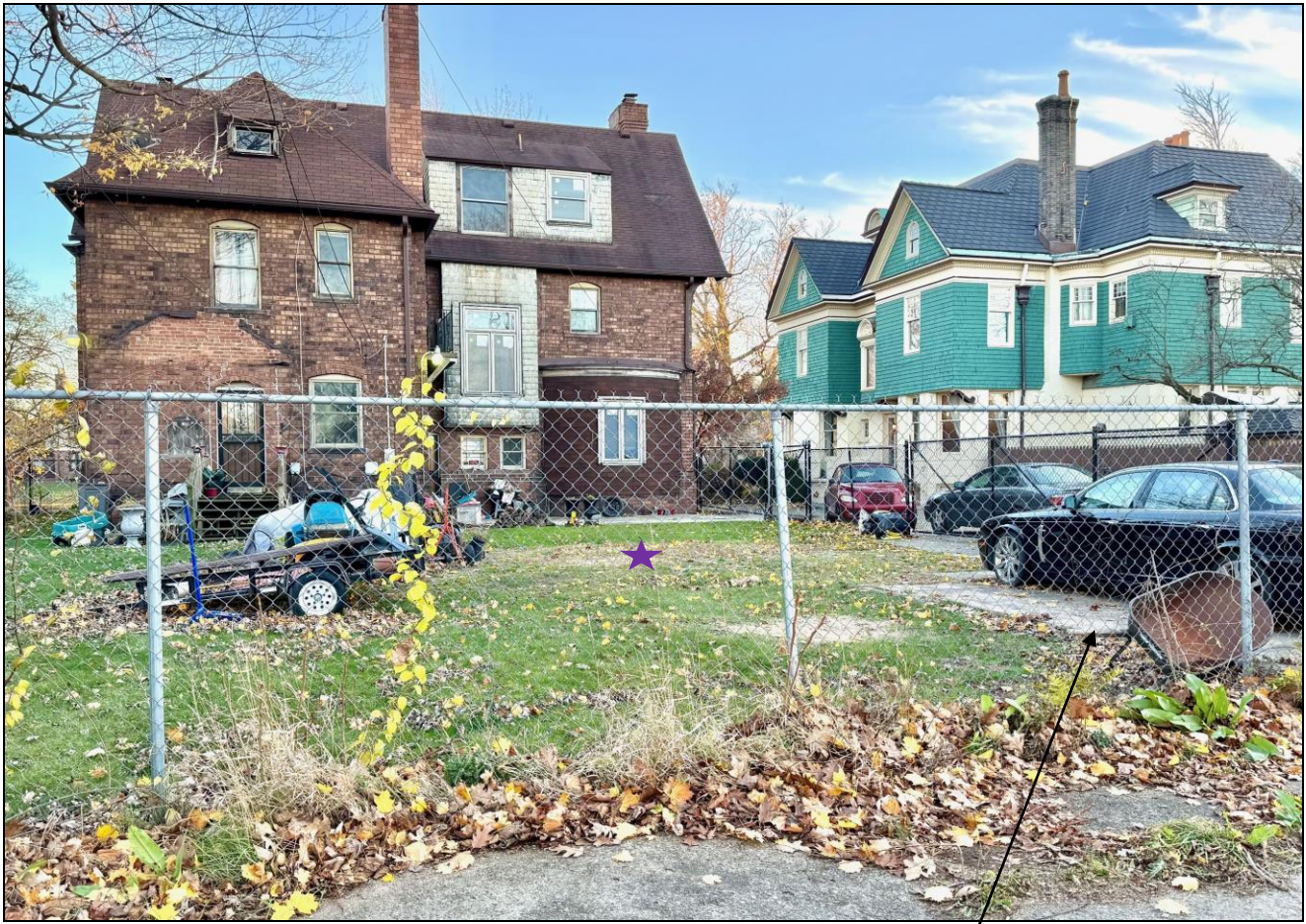
View of existing conditions at rear yard of 235 E. Boston Boulevard looking southwest from public alley. The historic garage was demolished at an unknown time; the concrete pad remains in place at the northwest rear corner of the lot. An overgrown concrete pad is near the center of the rear yard (★). Staff photo, November 26, 2024.
