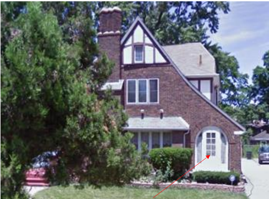
Google Streetview, 2013. Note that historic wood door with leaded glass sidelites are present
