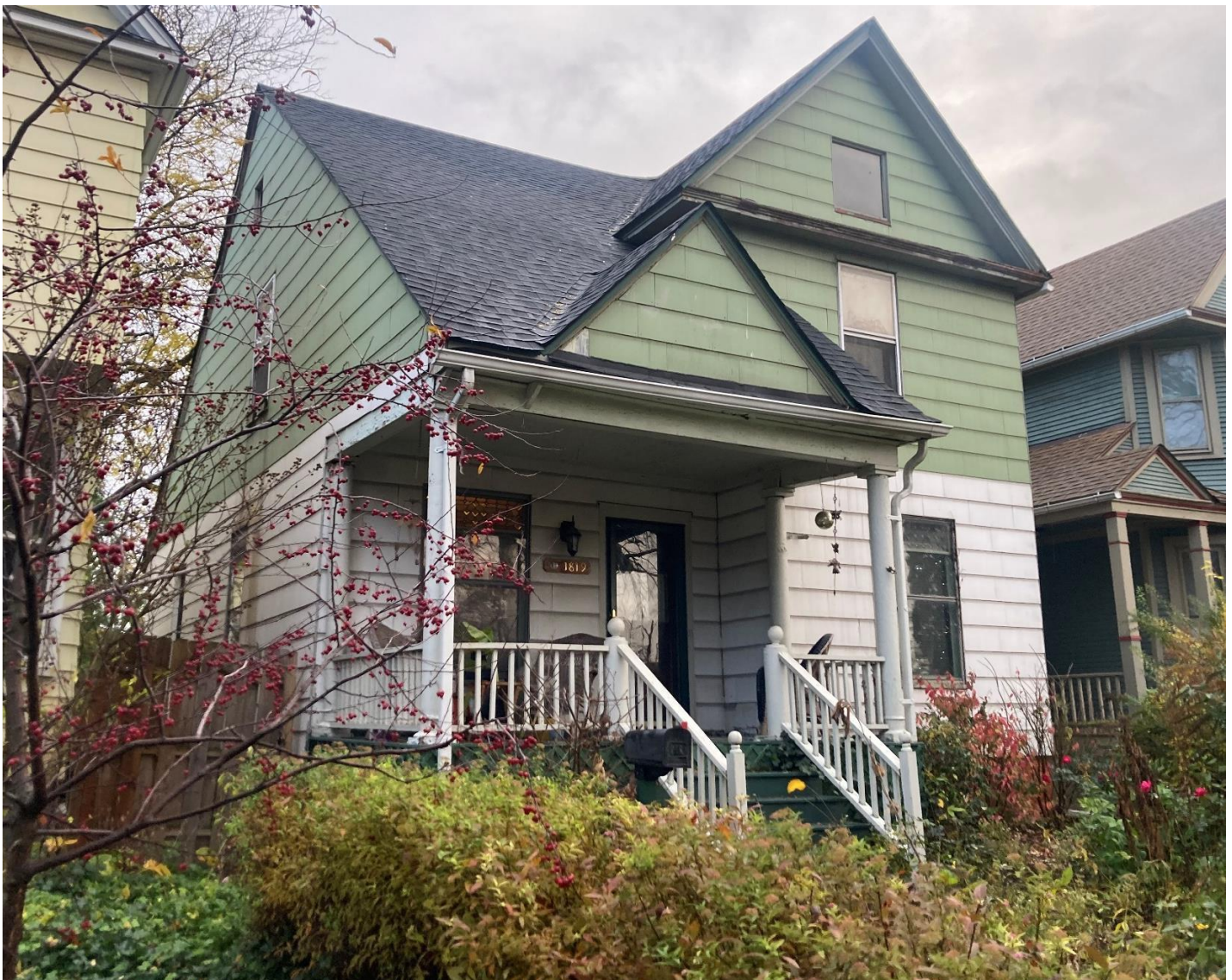
1819 Leverette, Staff photo of current conditions. Photo taken on 11/20/2024
