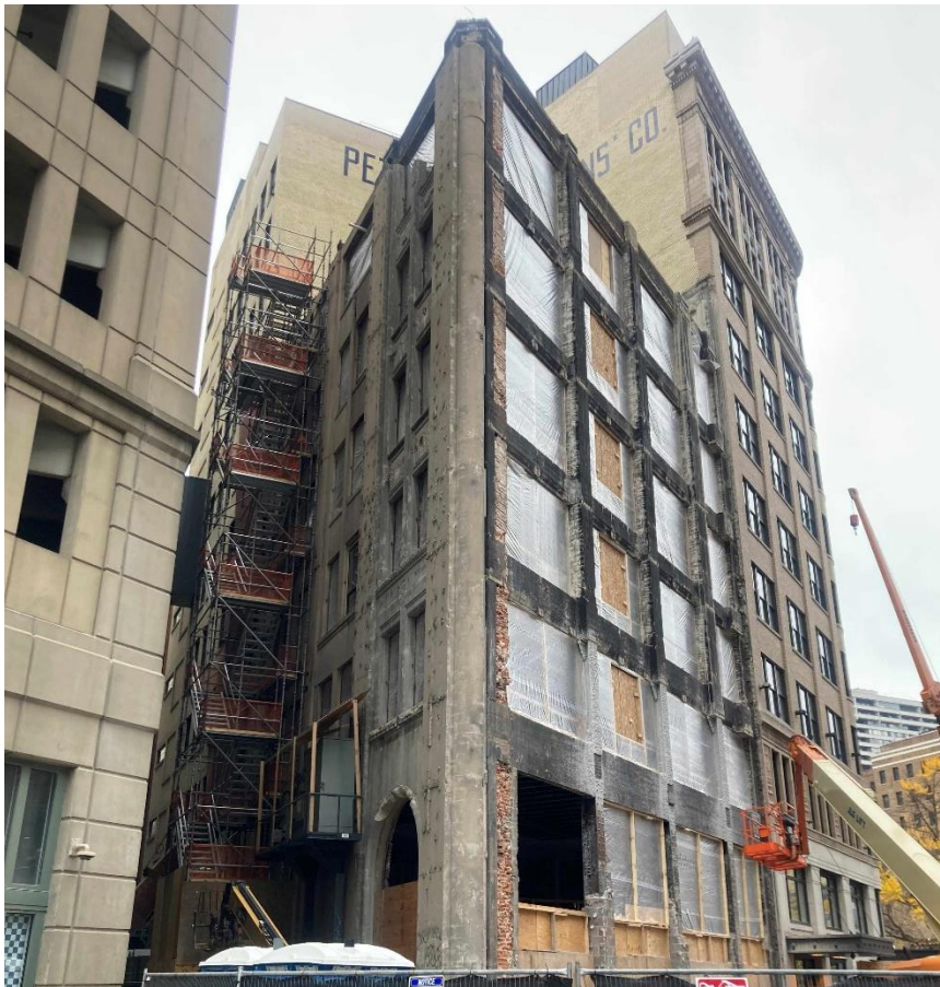
1133 Griswold, current conditions. Photo by HDC staff taken on 11/25/2024
