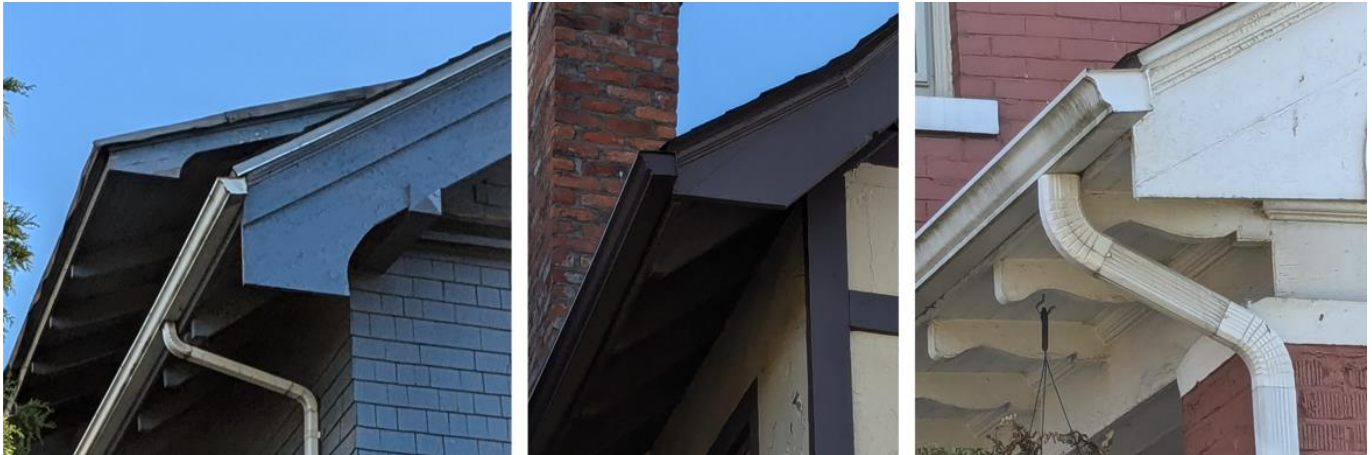
Examples of other Boston-Edison houses showing exposed vergeboards, beams, and rafter ends. Obscuring these features with soffit panels would not be appropriate. The use of a narrow fascia board and gutters that do not obscure these features is appropriate. November 2024 photos by staff.
