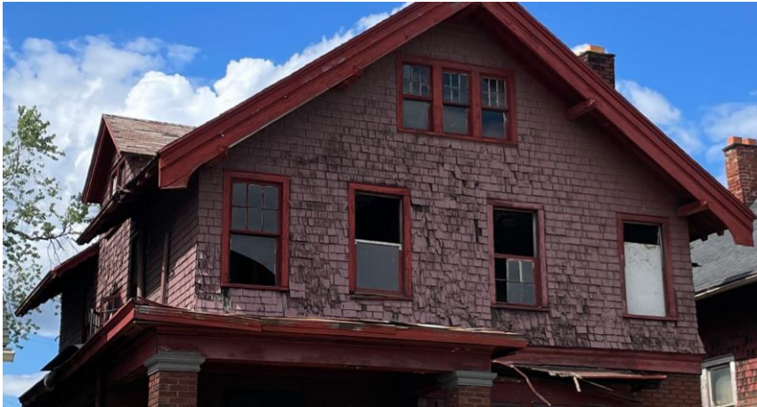
August 29, 2022, staff photo showing window removal.
