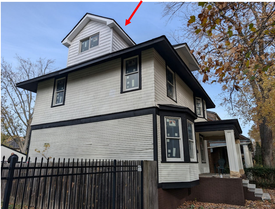
View of 708 Pallister, looking northeast. Note replacement windows in all openings, and the large gable-roofed dormer facing west, with incompatible sliding window, which reorients the emphasis from the front facade. Note also the apparent difference in color tone between the factory "white" of the dormer and the correct "yellowish white" color of main house. Staff photo, November 13, 2024.
