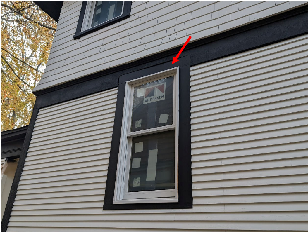
View of 708 Pallister, view of west (side) wall. This window opening was not approved, and trespasses into the historic wooden "belt band" between the 1 st and 2 nd stories (red arrow). The framing is incompatible in width, inset, and material (imitation "wood grain" composite). Staff photo, November 13, 2024.
