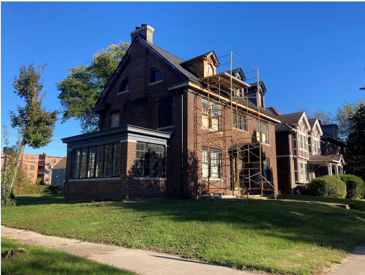
Current condition, staff photo taken on 10/16/2024
